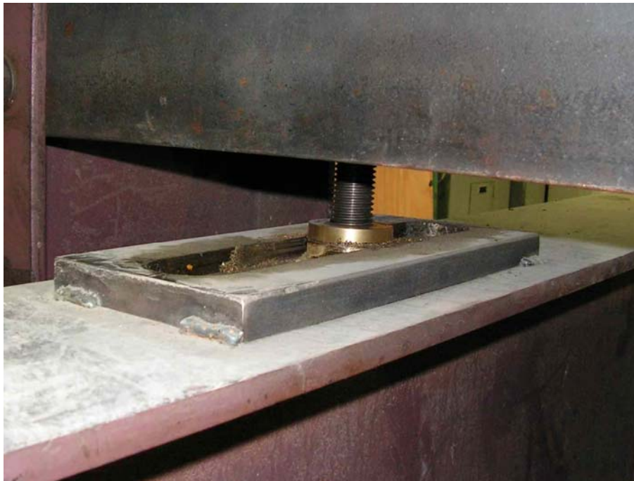
Figure C-4 Leveling Bolt Improvements, Lowered Position
