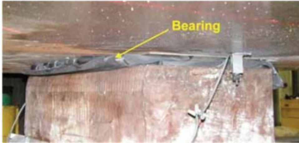
a) Bearing Prior to Removal from Test Frame
