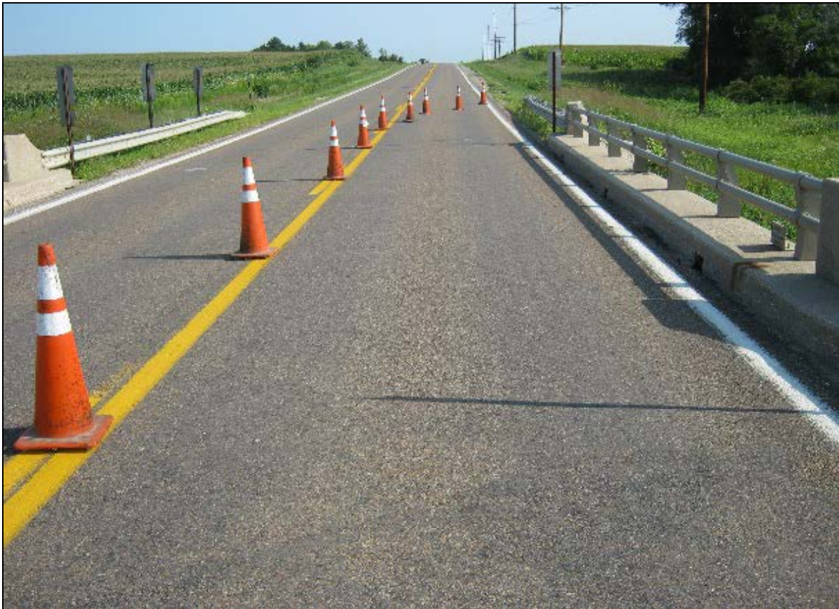
FIGURE 33 Photograph of Nebraska Bridge Deck 3.
