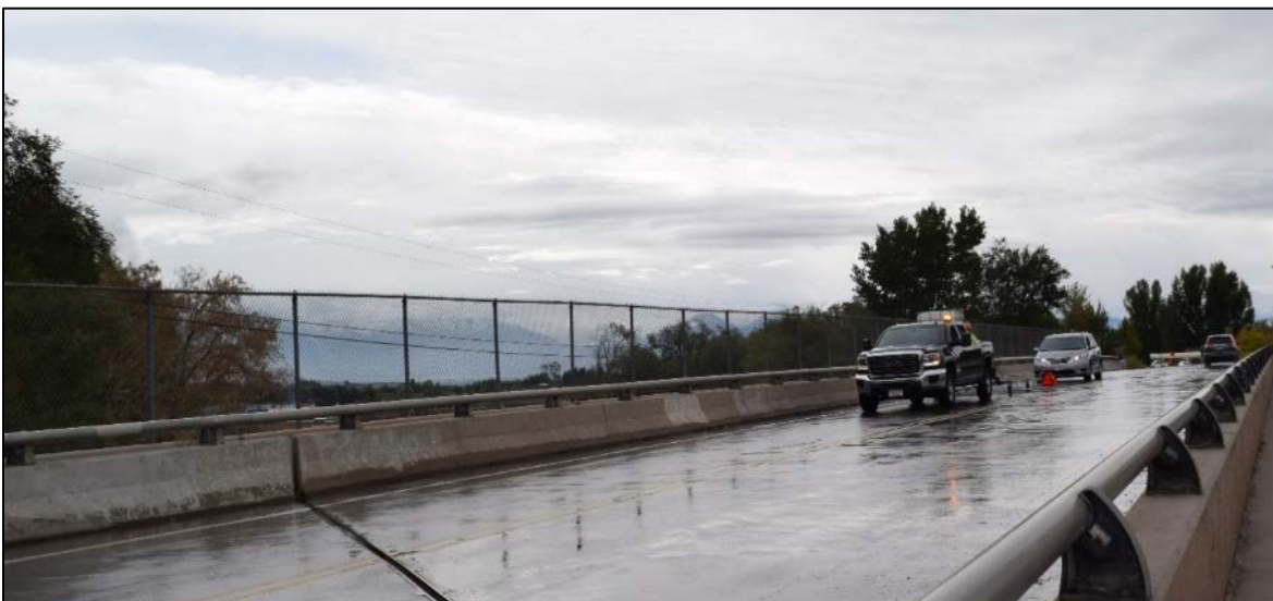
FIGURE 35 Photograph of VEI scanning on Utah Bridge Deck 1.
