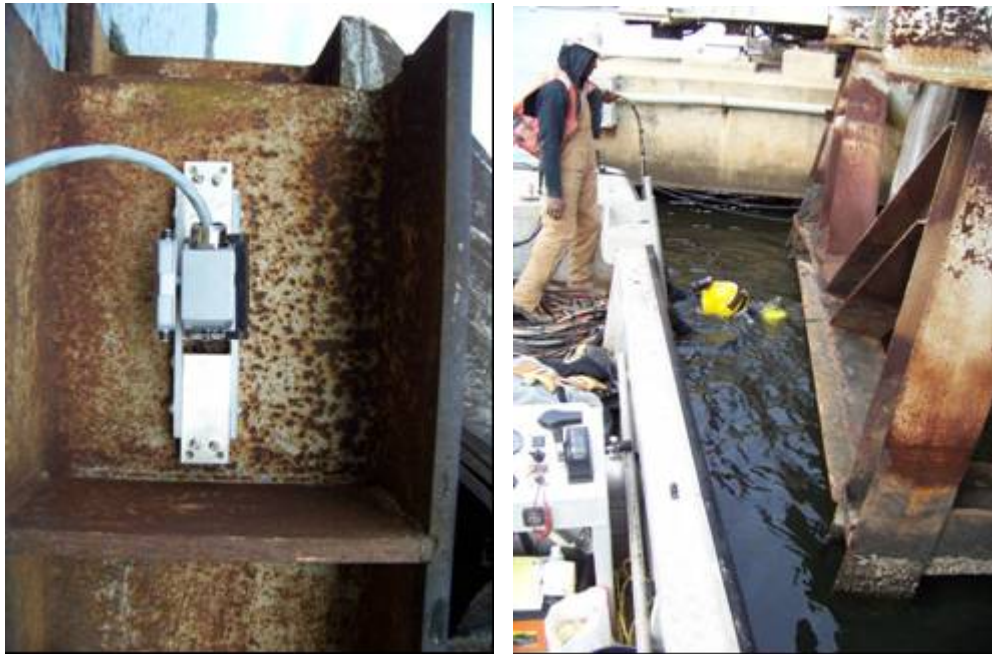
FIGURE 17 Field Testing in New Bern, NC
