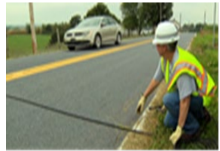
FIGURE 1 Road Tube Installation
