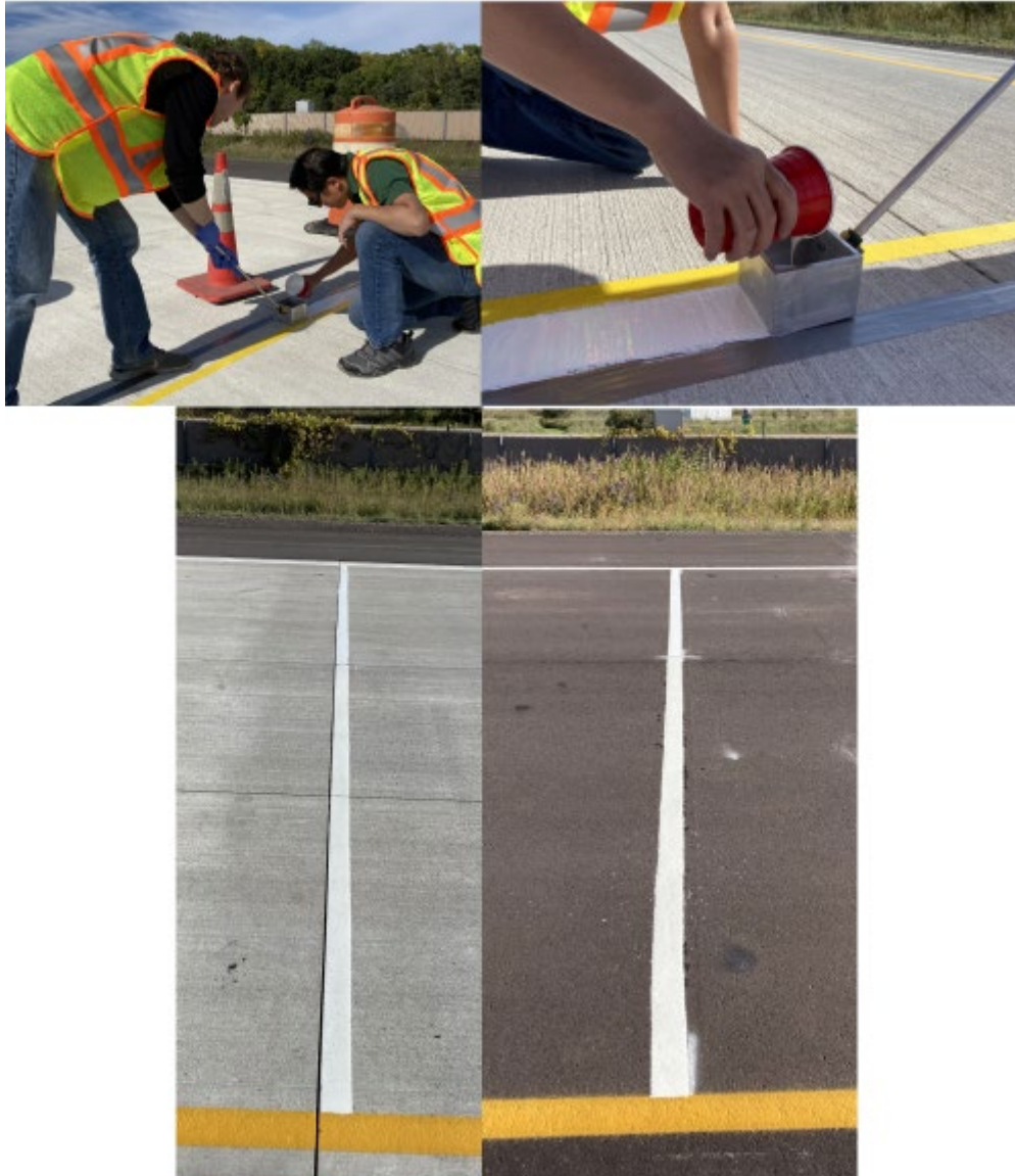
FIGURE 48. Application of the marking at the MnROAD I-94 test section.
