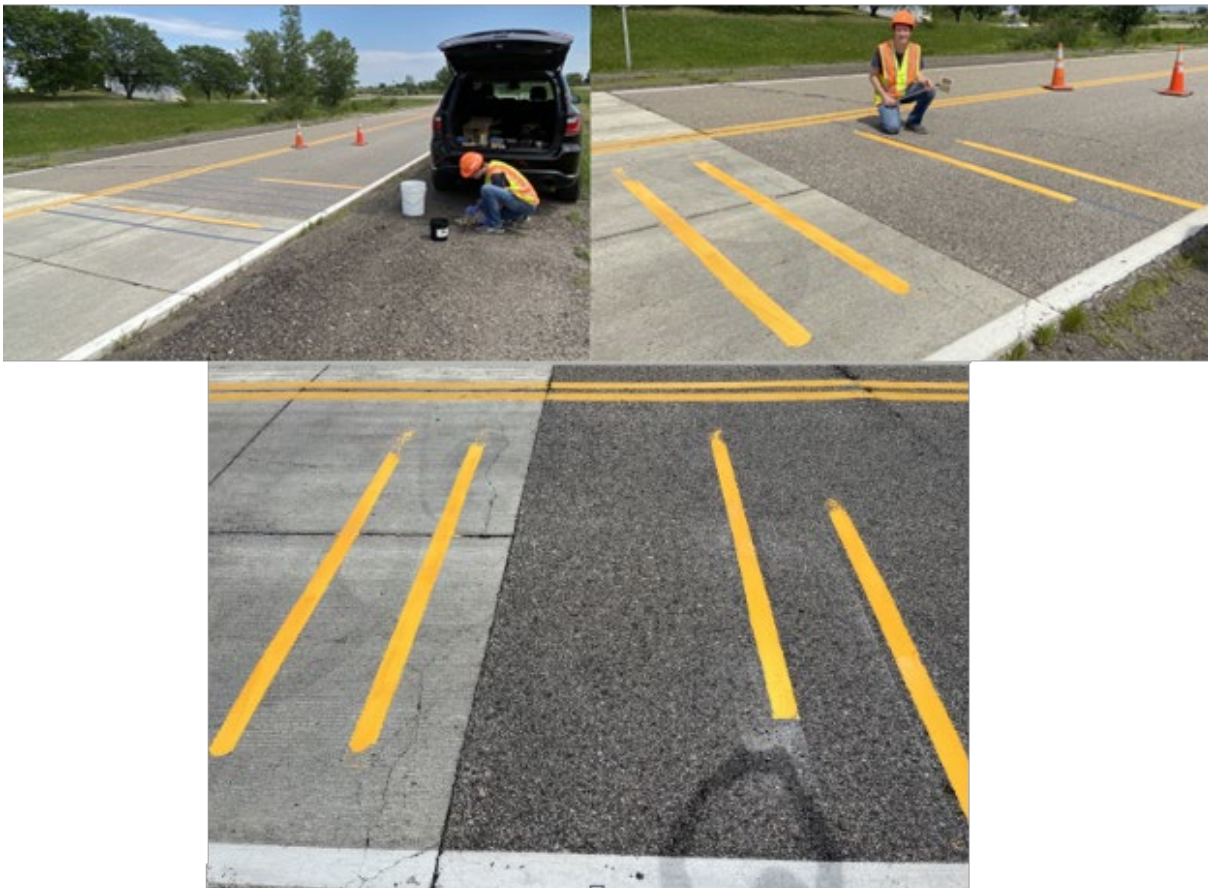
FIGURE 47. Pavement application on MnROAD test track.
