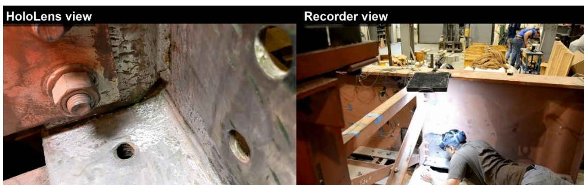
Figure 63 Inspector collecting a video for crack detection
