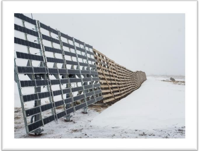
Solar snow fence in solar tracking operation (left) and snow fence position (right).
