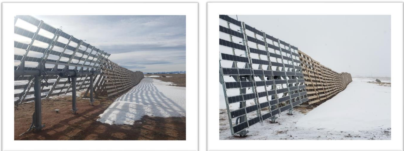
FIGURE 31: Solar snow fence in solar tracking operation (left) and snow fence position (right).
