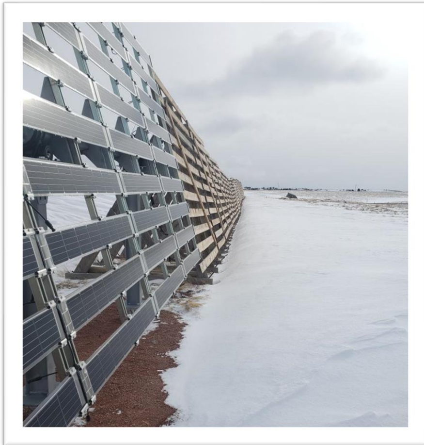
FIGURE 2: 12 foot (3.6 m) high solar snow fence co-located with a wooden snow fence.
