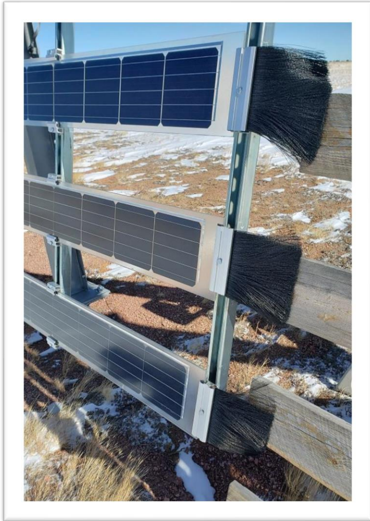
FIGURE 23: End-brushes in contact with the wooden planks of the co-located snow fence.
