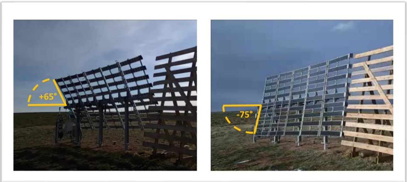
FIGURE 7: Solar snow fence solar tracking range-of-motion.
