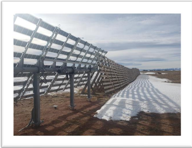
Solar snow fence in solar tracking operation (left) and snow fence position (right).
