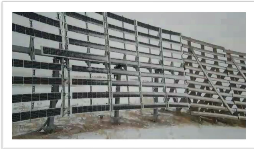
Figure 27: Wind-driven snow accumulating on the front side of both snow fences.
