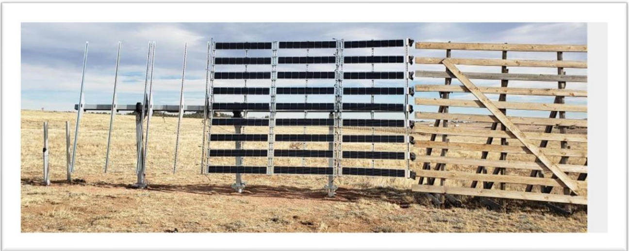
FIGURE 5: Partially assembled solar snow fence with monofacial solar panels attached.
