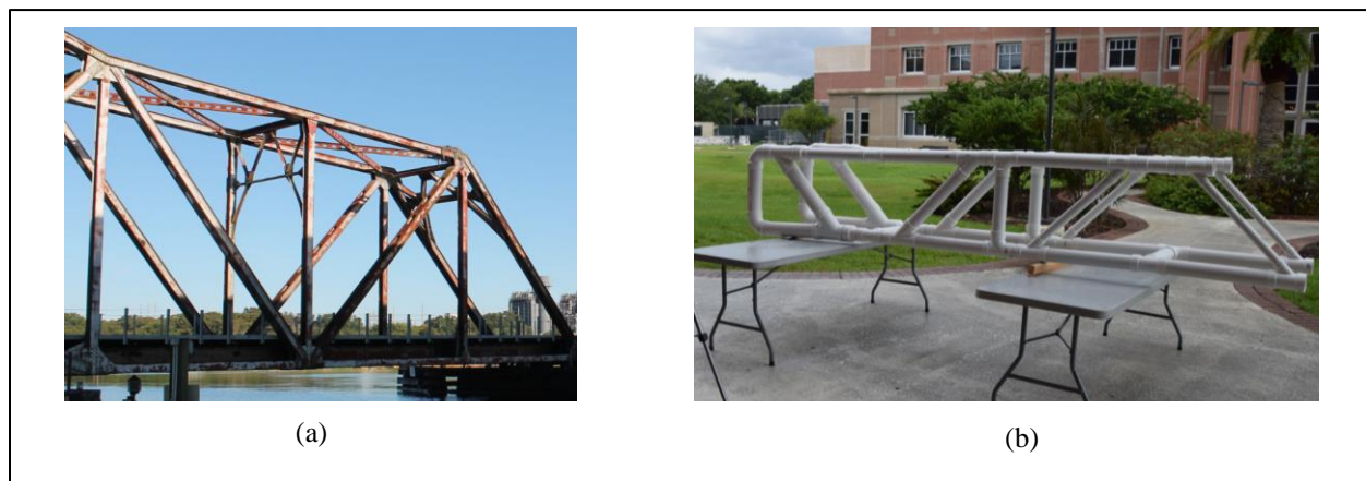
Figure 5-2 (a) Real-life railroad bridge (b) PVC bridge structure for controlled experiments.
