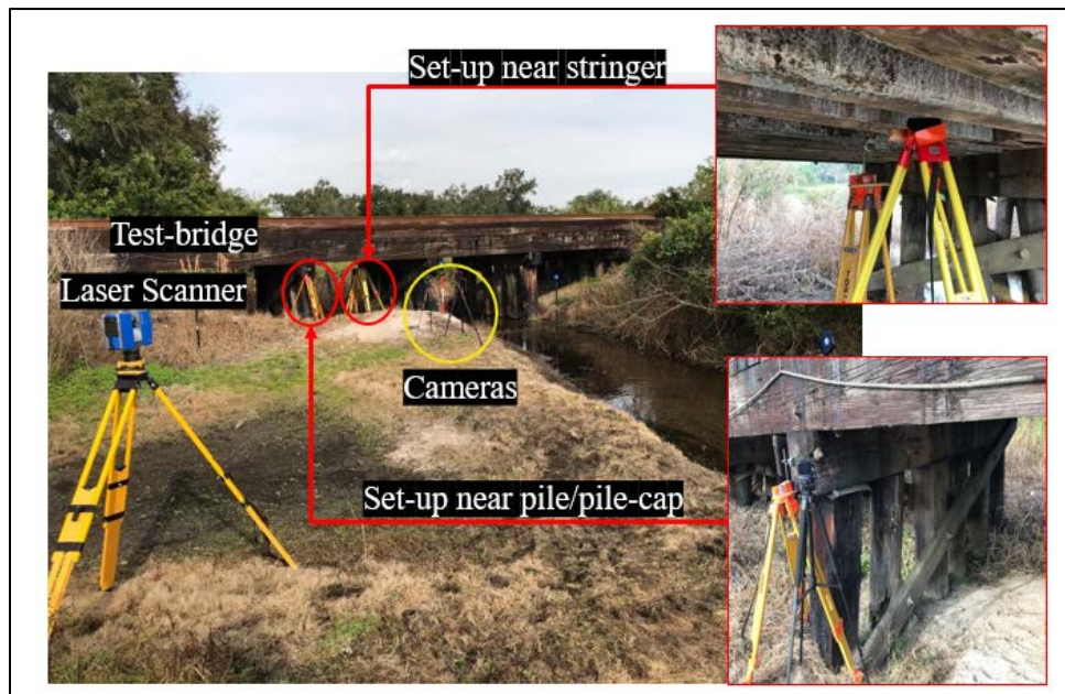
FIGURE 9. Field Test Set-up for Site SX 878.8
