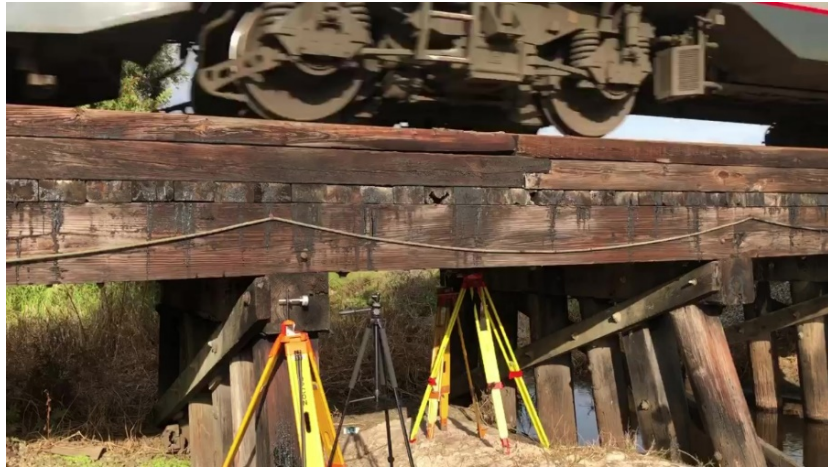
FIGURE 10. Amtrak passenger car axles used for dynamic load testing in SX 878.8
