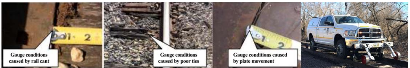
Figure 42. Track displacement checks and geometric car.
