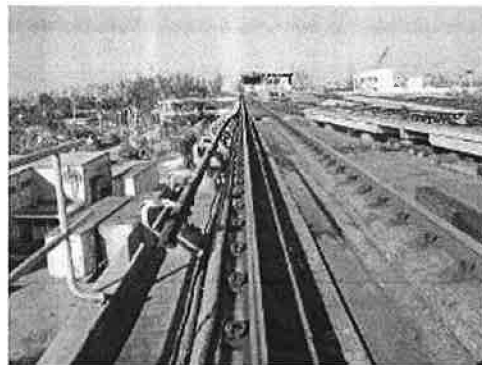
Fig 5. Weakened cover board blown off by Hurricane Wilma, Miami, October 2005
