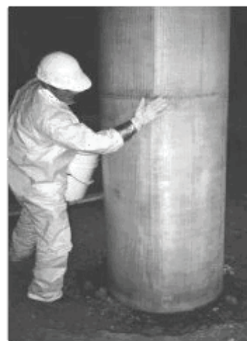
Pier concrete column after wrapping.
