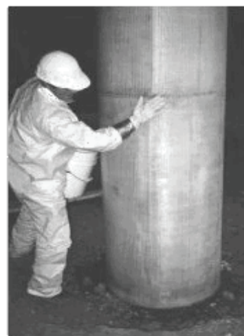
Pier concrete column after wrapping.
