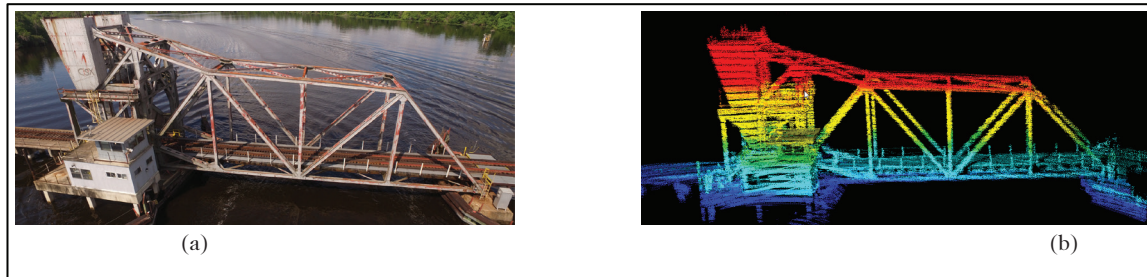
Figure 3: (a) CSX's railroad drawbridge; (b) 3D model of drawbridge from LiDAR data.
