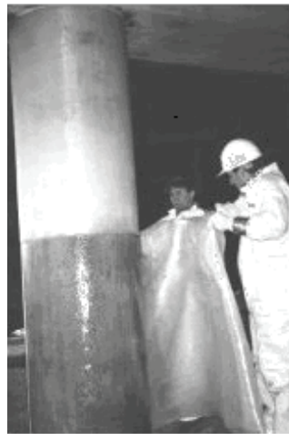
Application of fiber composite wrap on Pond Creek Bridge.
