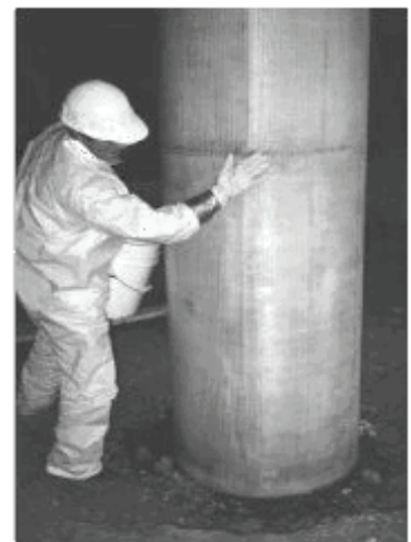
Pier concrete column after wrapping.
