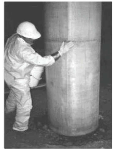
Pier concrete column after wrapping.
