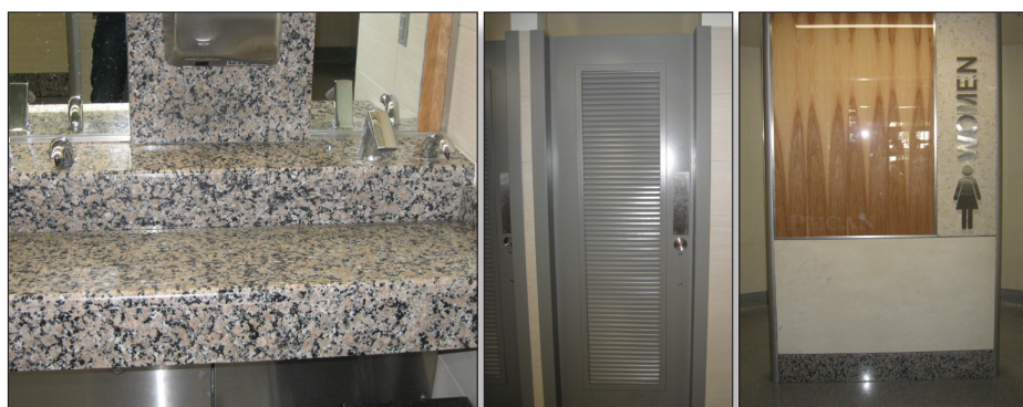
Above: Remodeling improvements to the terminal restrooms at Austin–Bergstrom International Airport (ABIA) include solid surface sink basins with touch-free faucets and hand dryers (left photo), metal stall doors with full louvers (center photo), and updated wall treatments featuring locally available limestone and pecan wood materials. ABIA staff used ACRP Report 130 to help guide their restroom redesign and remodeling plans. Photos courtesy of ABIA.
