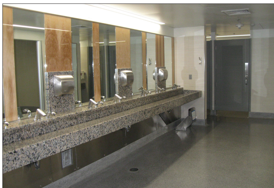
Above: Renovated terminal restroom at Austin-Bergstrom International Airport (ABIA). Airport staff referenced ACRP Report 130 to improve remodeling plans. The renovation features contemporary design materials including granite sink basins and countertops, wood veneer and stainless steel wall panels, and LED lighting strips. Photo courtesy of ABIA.
