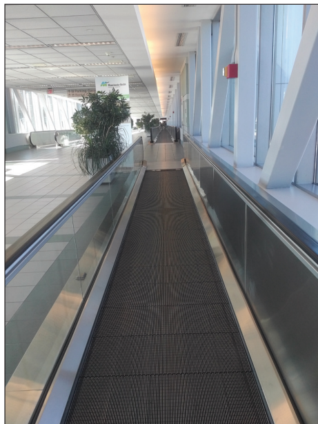
Above: Moving walkways at Manchester-Boston Regional Airport (MHT). Staff at MHT referenced ACRP Report 117 in the decision to install lower energy motors, LED lighting, and motion detection switches on moving walkways to reduce energy use at the airport. Photos courtesy of MHT.
