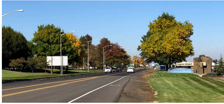
Figure 2: Entrance to Eugene Airport
