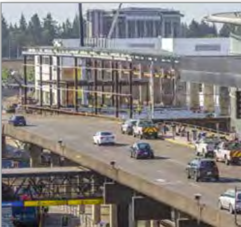
Construction begins on the new IAF in 2018 (Source: Port of Seattle).
