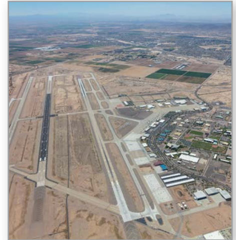
Aerial view of Phoenix–Mesa Gateway Airport (Source: Margi Evanson, Phoenix–Mesa Gateway Airport).
