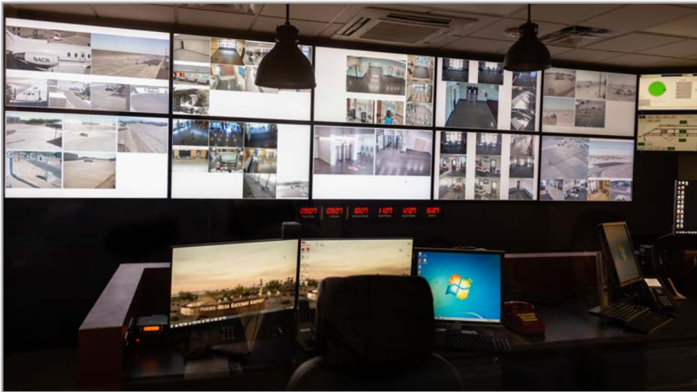
Redesigned ACC room at Phoenix–Mesa Gateway Airport with video wall (Source: Margi Evanson, Phoenix–Mesa Gateway Airport).
