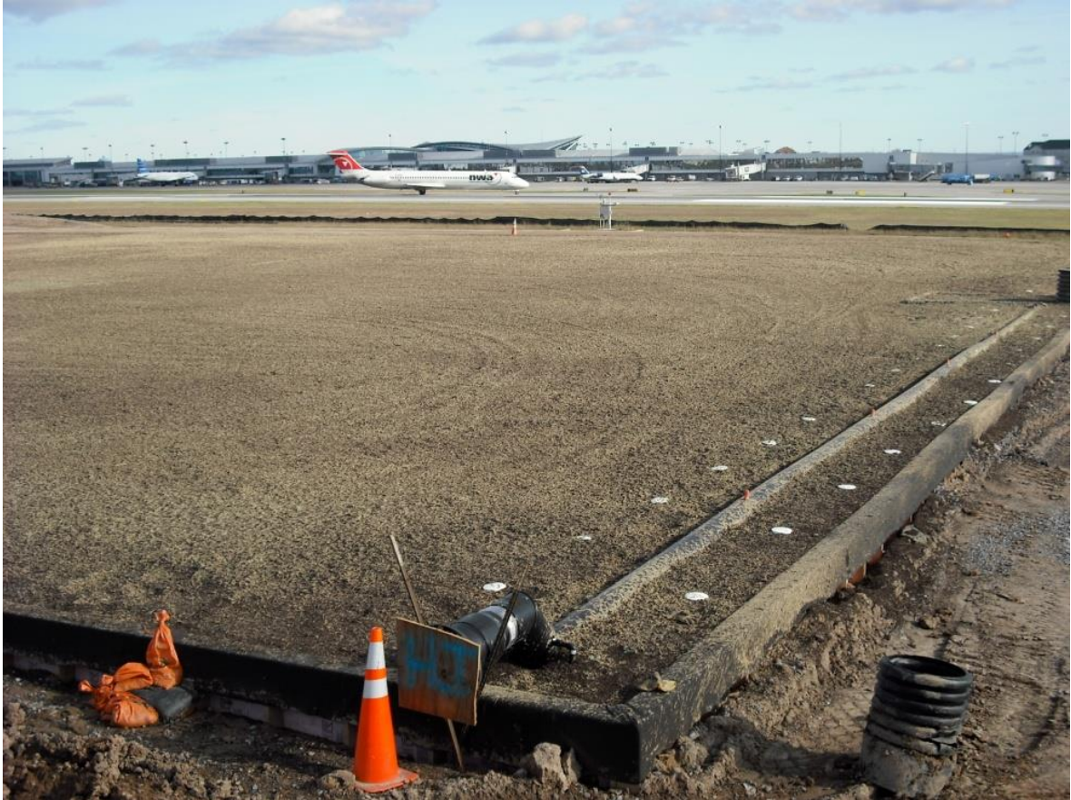
Figure 2. Aerated gravel bed at Buffalo Niagara International Airport (courtesy Mark Liner).
