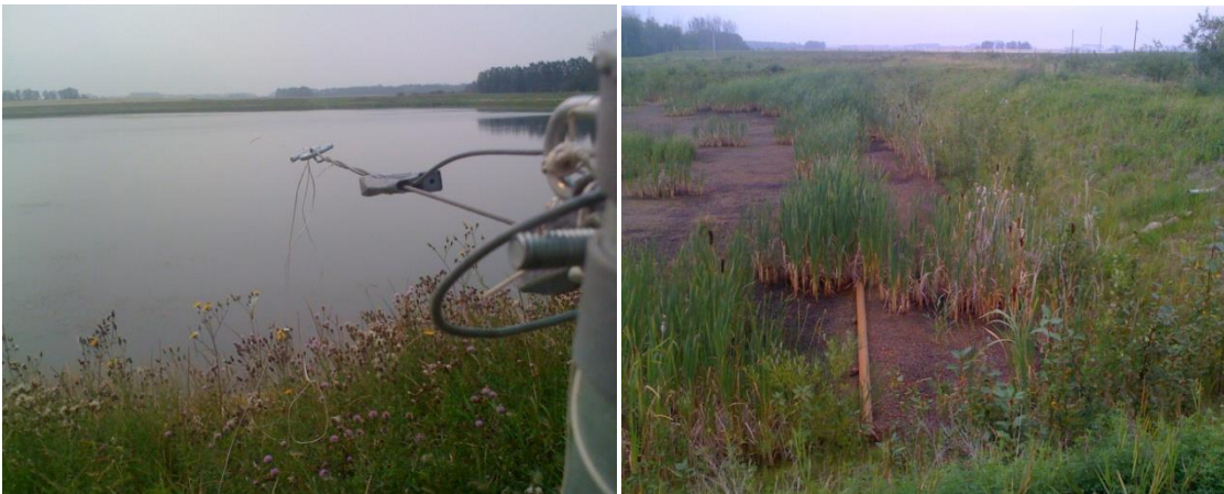
Figure 2. Facultative lagoon and treatment wetland at Edmonton International Airport
