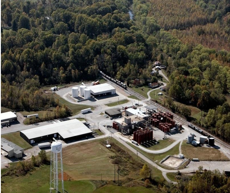
Figure 1. Private recycling facility in Troy, Indiana.
