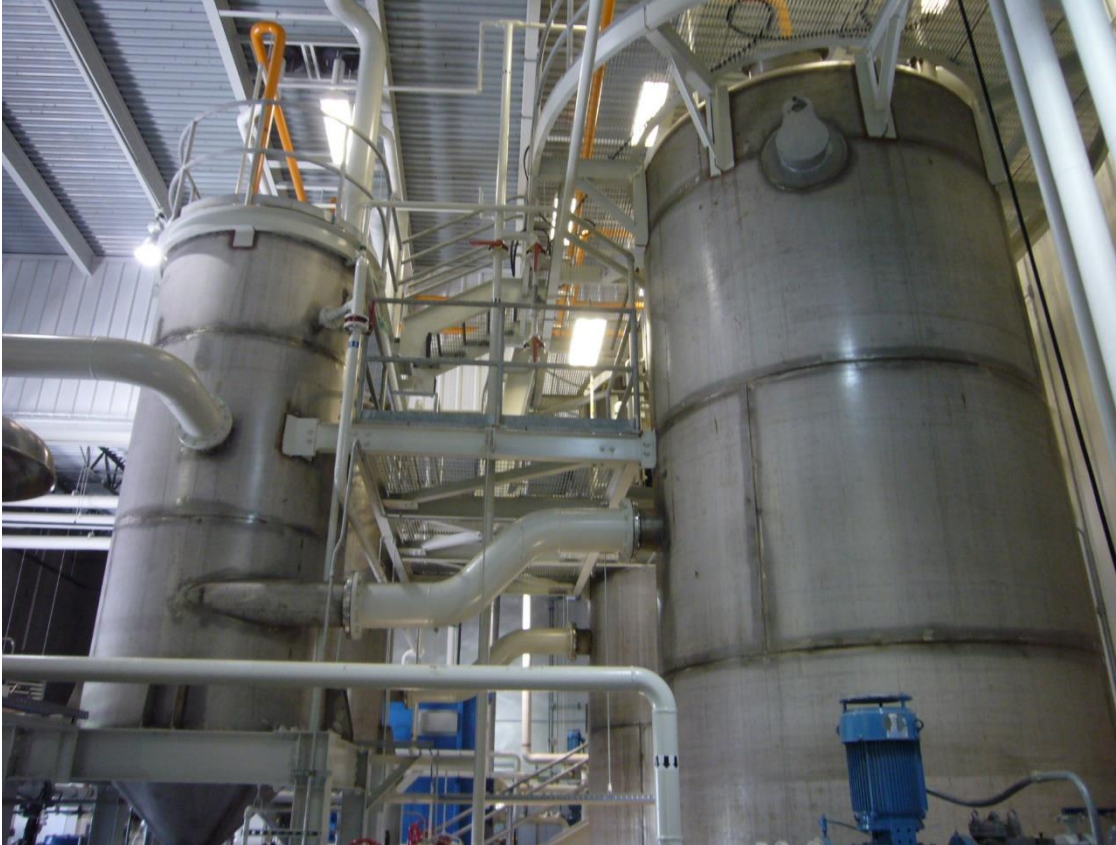
Figure 2. Biological reactor units (at right) in the CAK AFBR system (courtesy of Gresham Smith).
