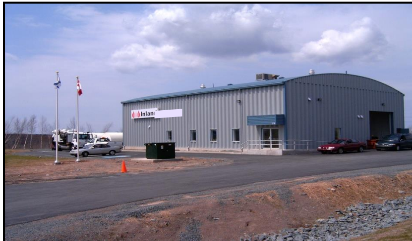
Figure 1. YHZ glycol recycling facility.
