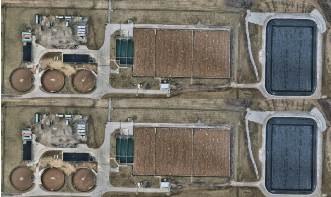
Figure 2. Aerial photo of CVG-activated sludge treatment system.
