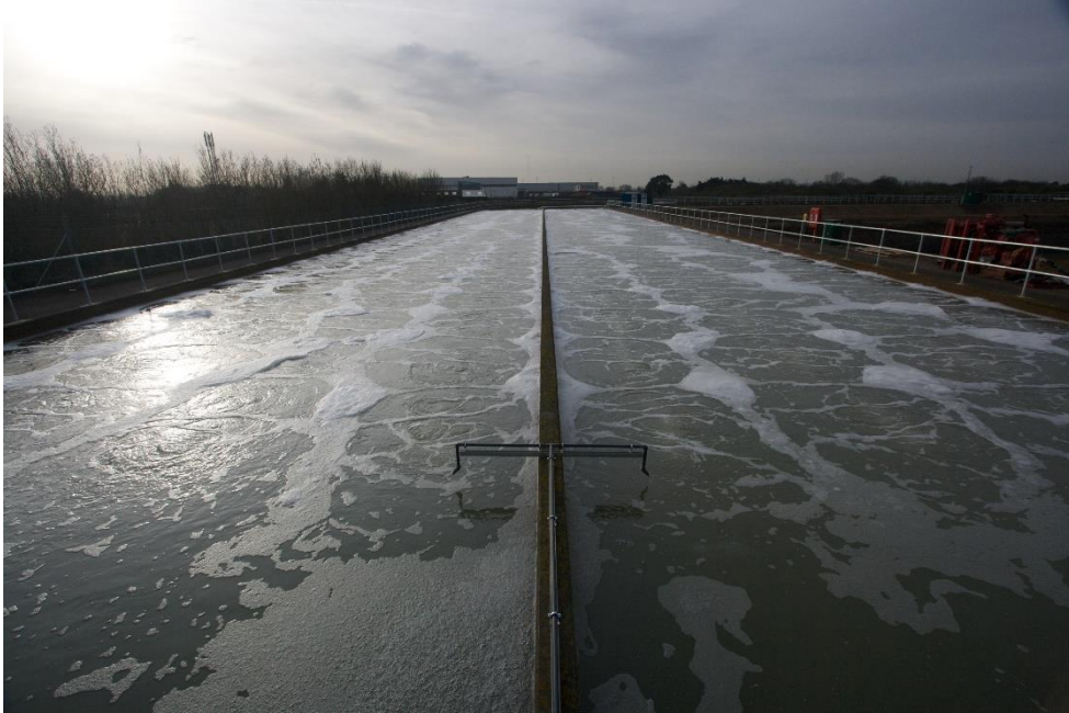
Figure 4. Complete mix aerated channel (courtesy of ARM Group LTD).
