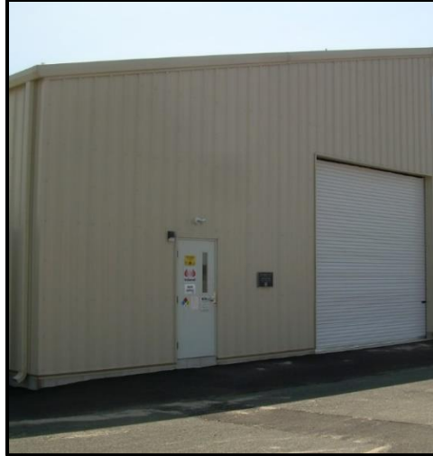
Figure 2. New Processing Building 2021.
