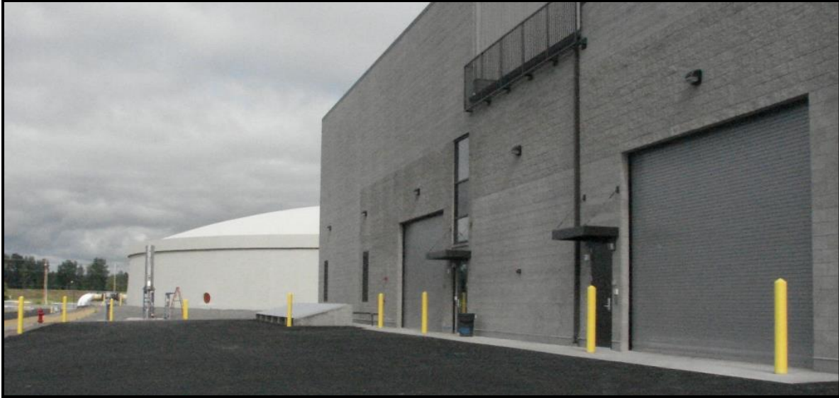
Figure 2. PDX on-site treatment facility site (courtesy Gresham Smith).
