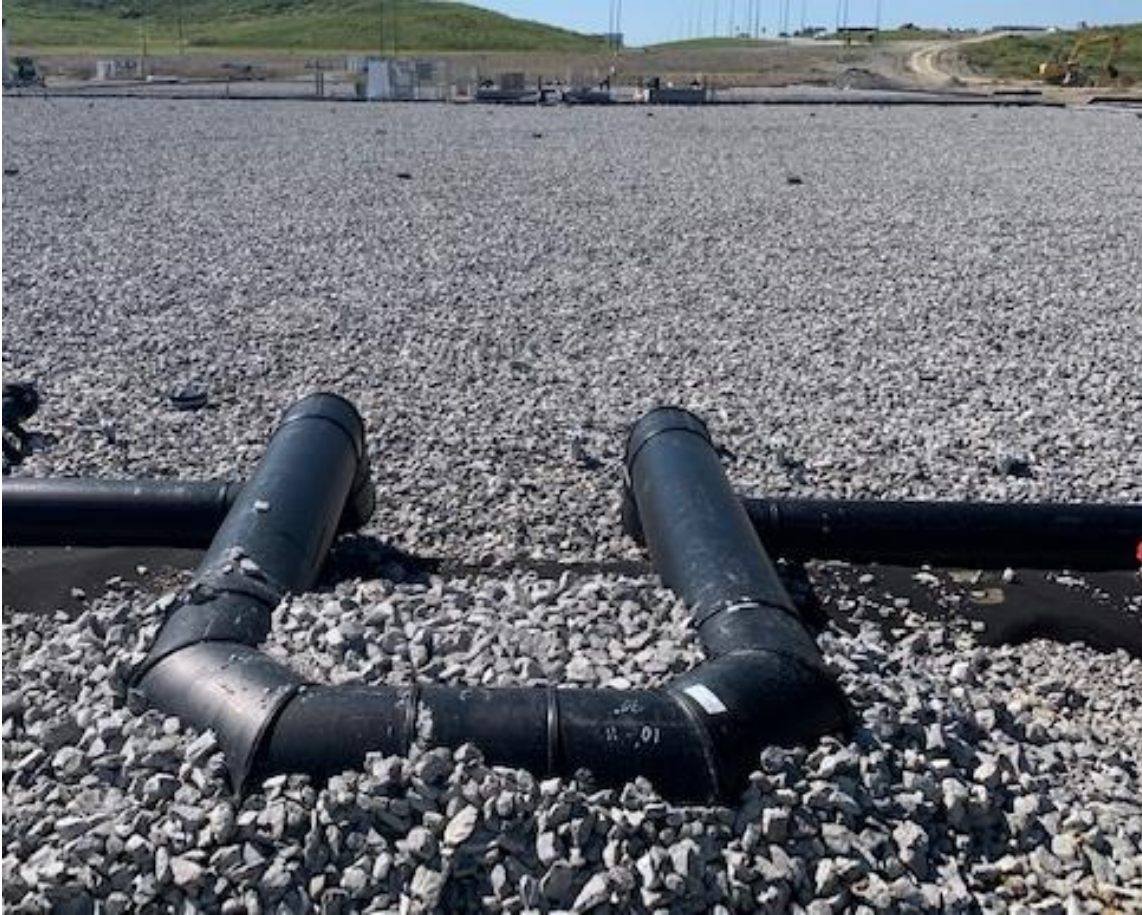
Figure 2. Aerated gravel bed cell.
