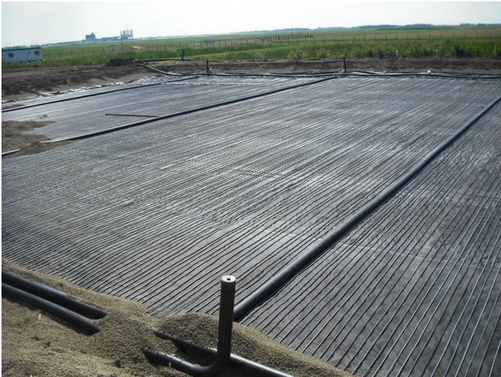
Figure 4. Installation of drain and aeration lines.
