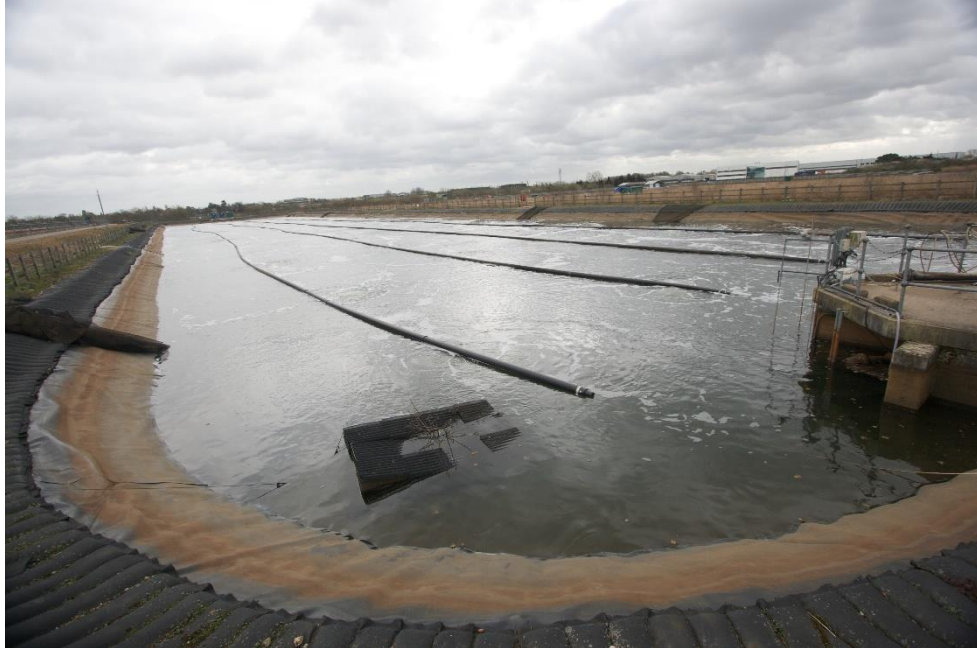
Figure 6. Partial mix lagoon (courtesy of Mark Liner).
