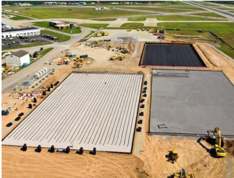
Figure 2. Construction of the BNIA aerated gravel bed.
