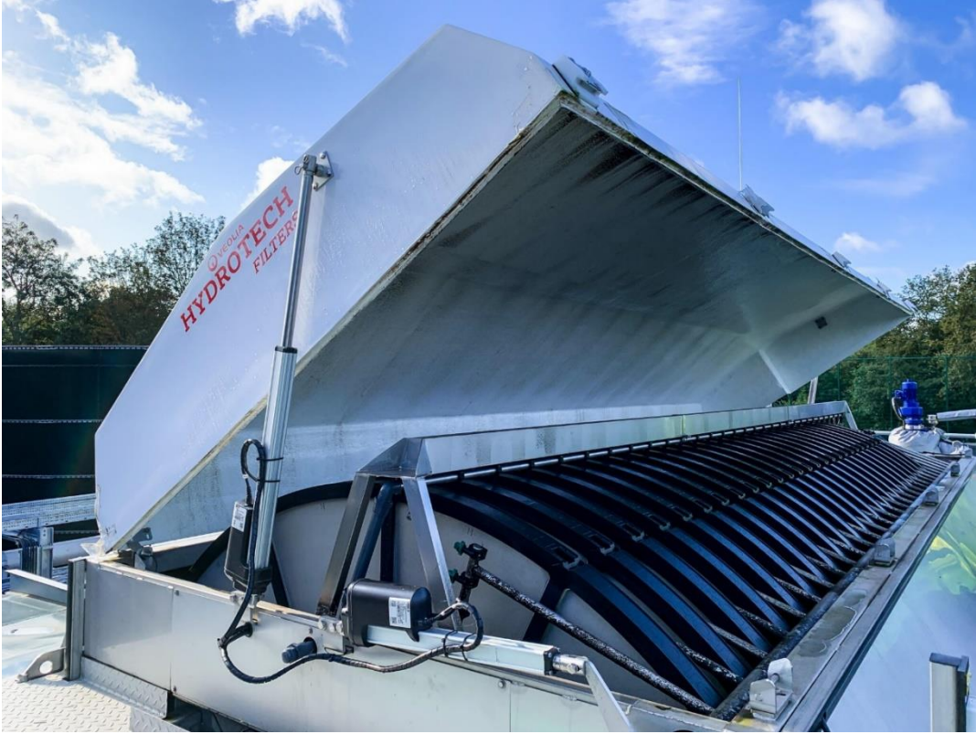
Figure 4. Disc filter (Airport World, 2021).
