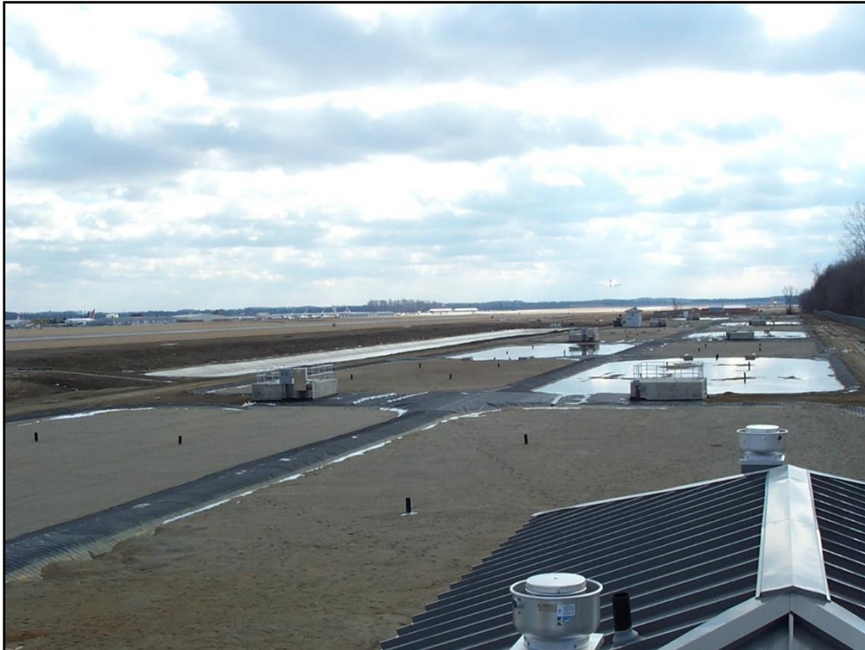
Figure 2. ILN reciprocating gravel bed system.
