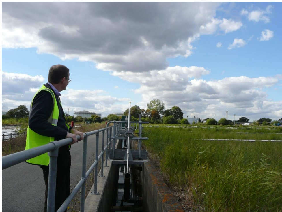
Figure 7. Aerated gravel beds (courtesy of ARM Group LTD).
