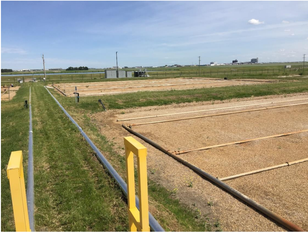
Figure 5. 2016 Upgrade with the terminal in the background (courtesy of M. Liner).
