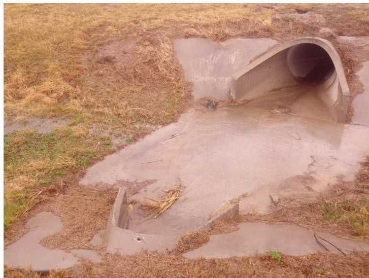
Figure H: Millard Airport Culvert
