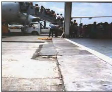
*Figure 1: FOD can be generated from broken pieces of pavement*
