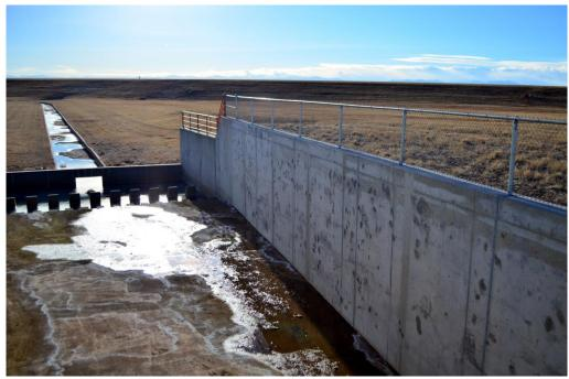
**Figure 6.1**. Box culvert at DIA receiving stormwater runoff from the west side of the airfield. The BOD loading rate and the flow rate of runoff entering Third Creek through sampling location D was estimated based on average rates of stormwater discharge sent to the Metro
