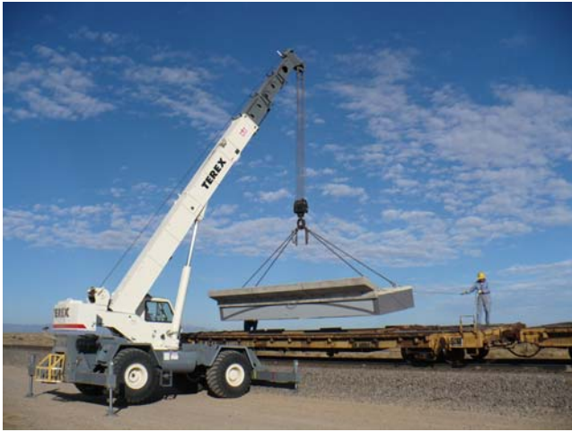
FIGURE 4.7 Unloading HCB Unit from Flatcar
