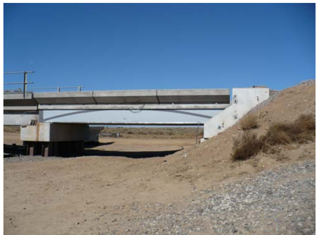
FIGURE 4.10 Complete HCB Span
