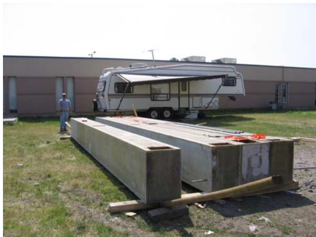
FIGURE 4.1 Tying Together HCB Units
