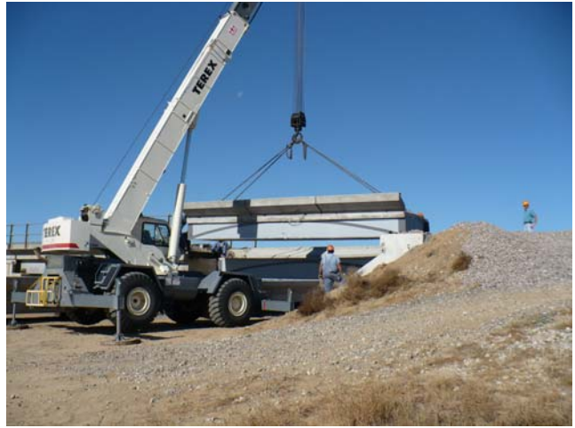
FIGURE 4.8 Setting HCB Unit on Bridge Substructure
