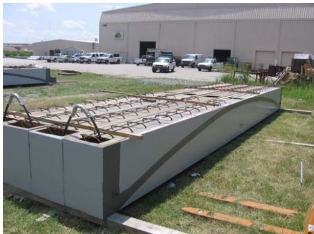
FIGURE 4.3 Four HCB Assembly without Concrete Reinforcing
