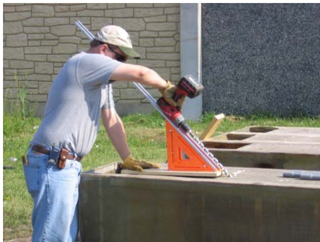
FIGURE 4.2 Drilling Holes for Shear Connectors
