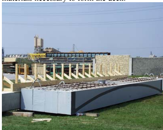
FIGURE 4.5 Forming Ballast Curbs and Deck
