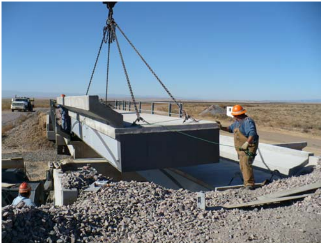
FIGURE 4.9 End View of HCB Unit During Erection
