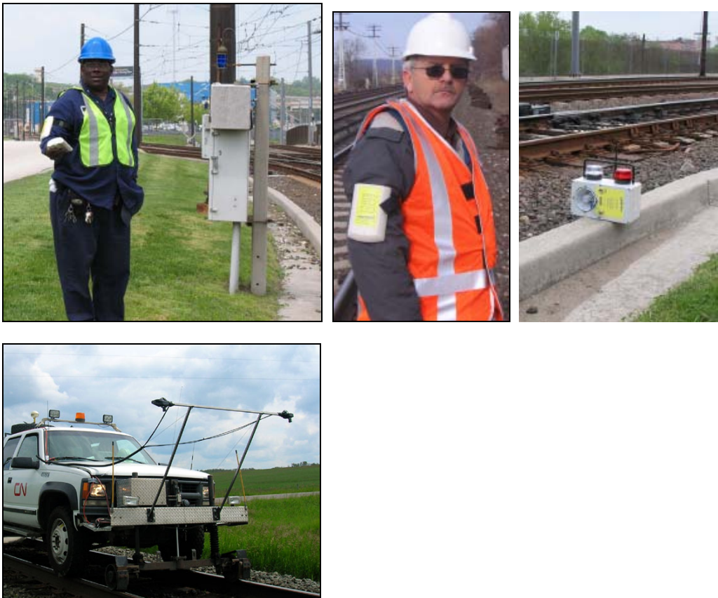
Figure 5 Flagger using the flagger supervisory device to activate the personal alert device, portable light/horn and rail vehicles.
