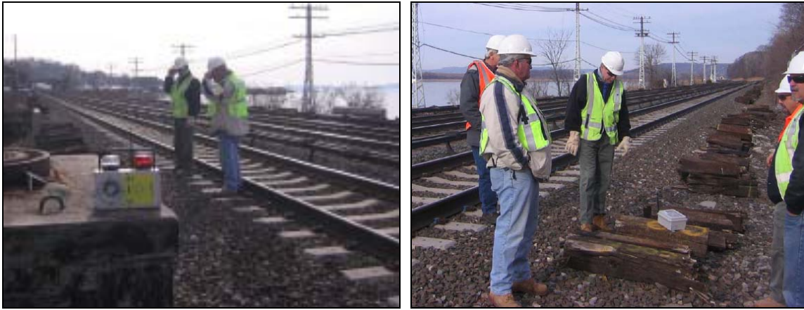
Figure 4 Portable light/horn unit place within the work zone.
