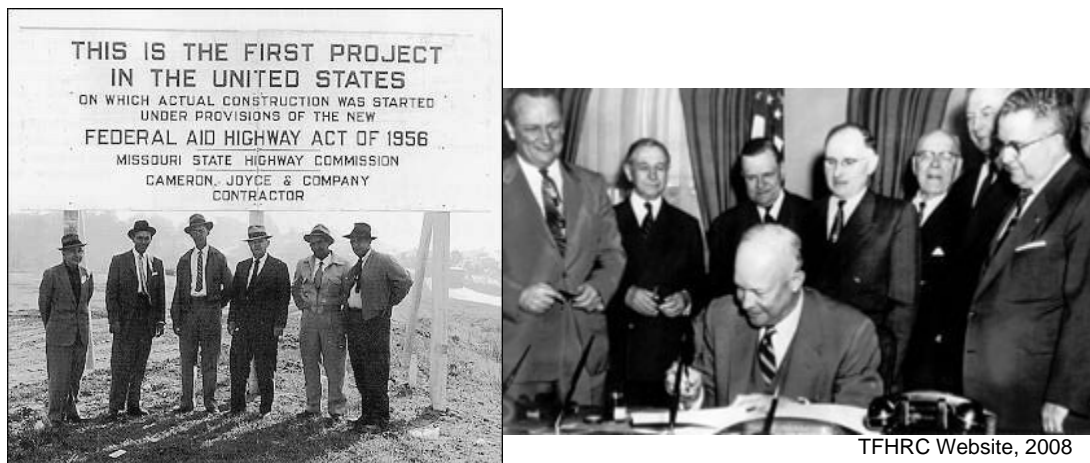
Figure 4. Federal Aid Highway Act Signed by President Eisenhower on June 29, 1956 to create today's interstate system (source FHWA Turner-Fairbank Highway Research Center website, 2008)
