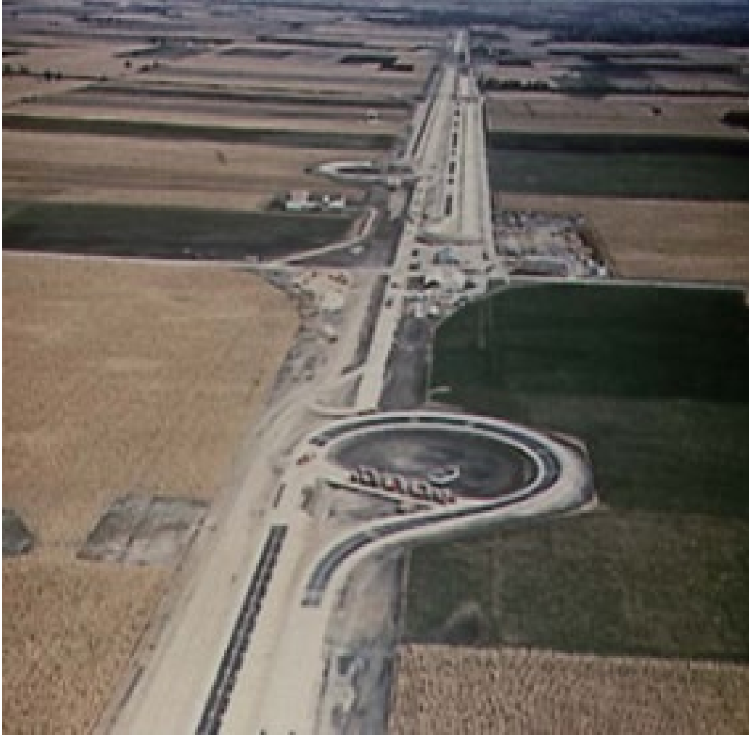
FIGURE 1 AASHO Road Test facility.
