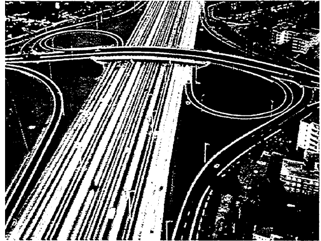
FIGURE 6 Partial Cloverleaf; Highway 401, Toronto, Canada
