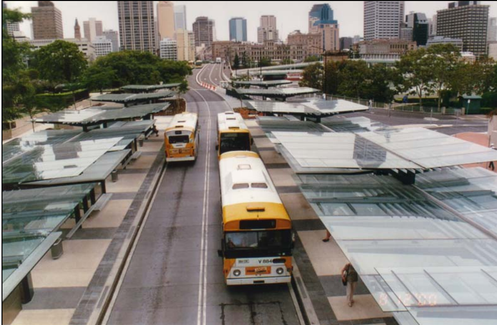
FIGURE 3 South–East busway at Southbank
