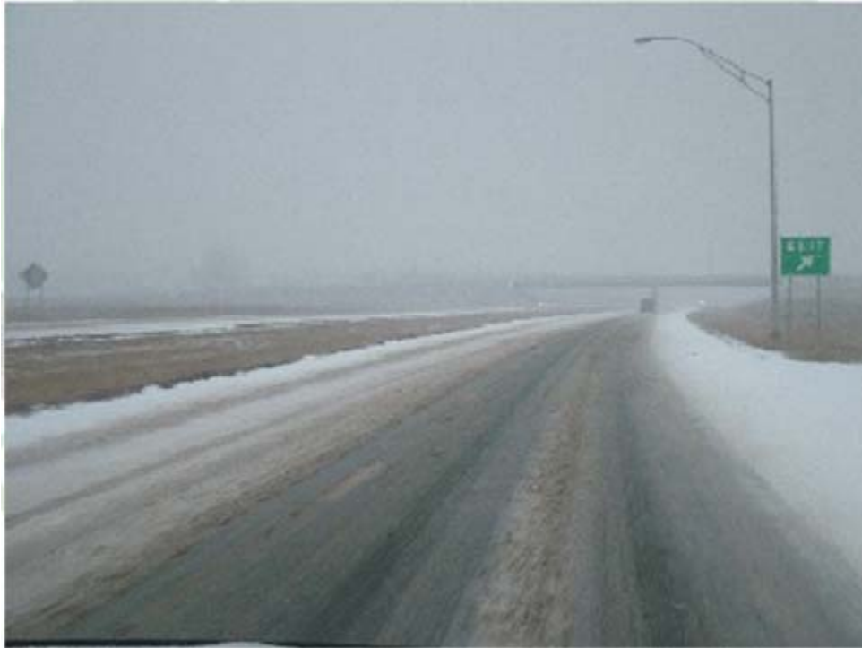
FIGURE 8 Photo of transition.
