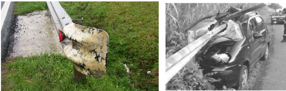
FIGURE 1 Unprotected barrier terminals (la Torre, 2011).
