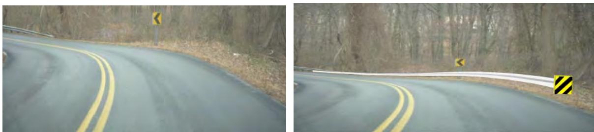
FIGURE 10 Potential solution by extending the guardrail.
