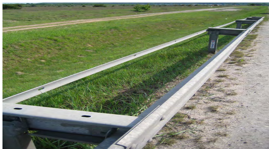
FIGURE 6 Inappropriate post spacings.
