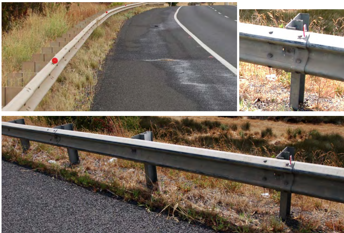
FIGURE 4 W-beam with Charlie post and block-out.
