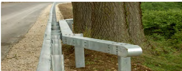
FIGURE 2 Stiffened barrier near a tree.
