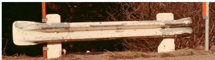
FIGURE 1 Typical fishtail or spoon terminal.
