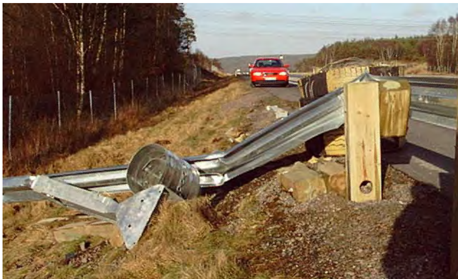
FIGURE 6 Energy-absorbing terminal.
