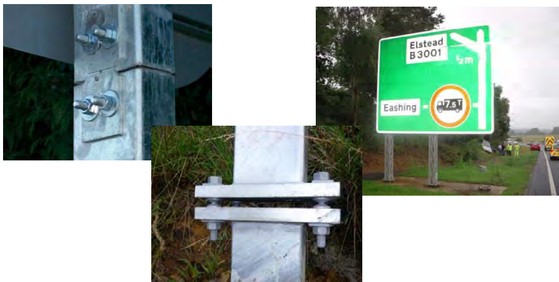
FIGURE 6 Passively safe support structures (la Torre, 2011).
