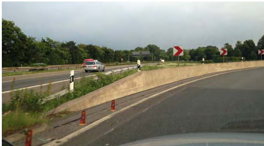
FIGURE 5 Use of ramped ends.
