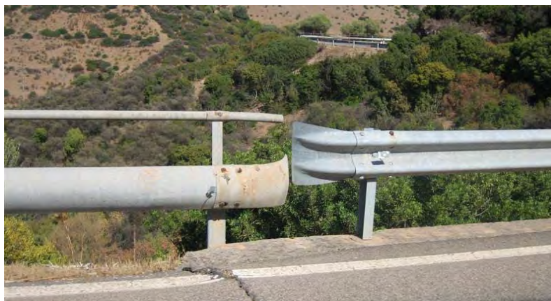
FIGURE 3 Barriers not connected.
