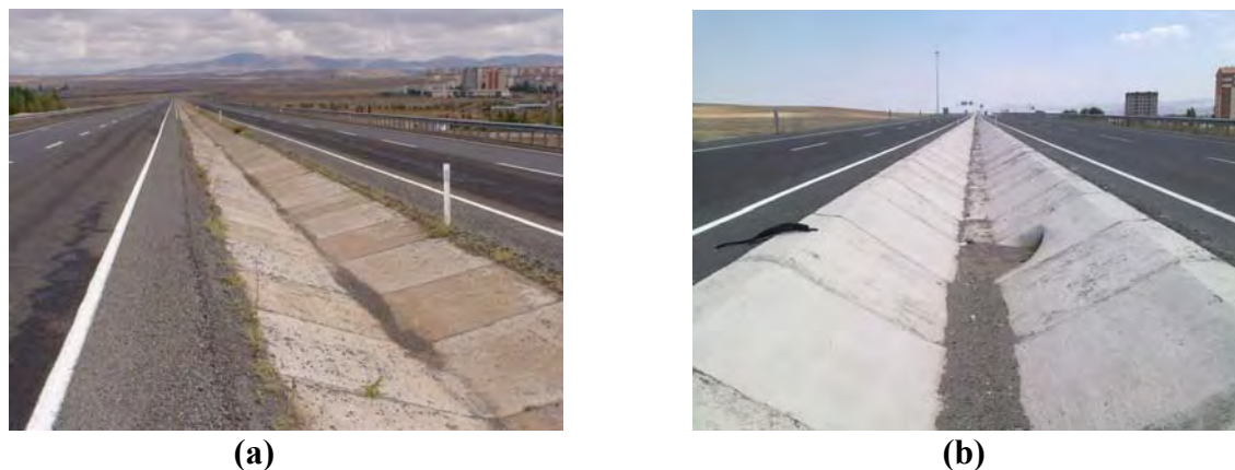
FIGURE 2 (a) Triangular-shaped ditch and (b) trapezoidal-shaped ditch at median.
