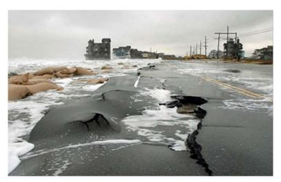
FIGURE 7 Pavement damage from surge and waves (13).
