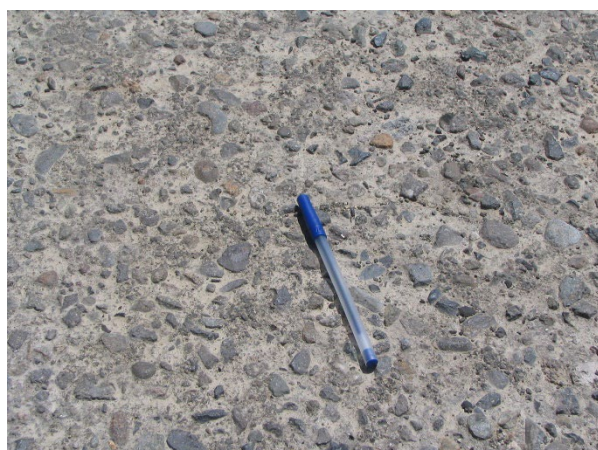
Figure 4.2 Oxidation and raveling (left), and bleeding (right) on asphalt concrete roads. (Image credit: RoadResource.org.)
