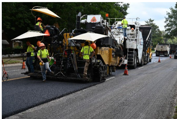
Figure 4.7 Application of a mill and fill (left) and a complete removal and replacement (right) on AC roads (image from A. Braham.)
