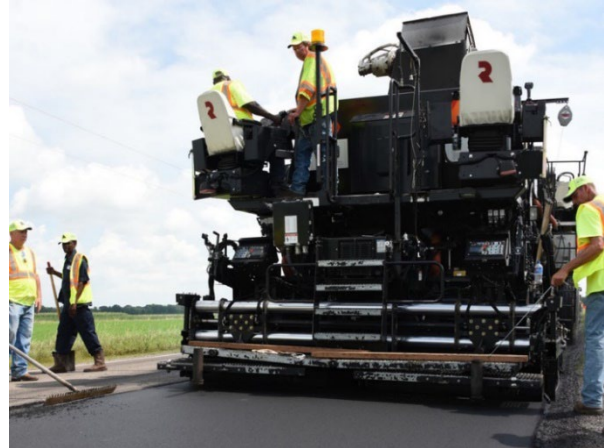
Figure 4.6 Application of a UTBWC (left) (Image credit: A. Braham) and a thin overlay (right) on AC roads (image from RoadResource.org).
