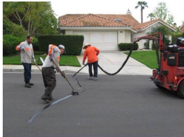
Figure 4.4 Application of a rejuvenating fog seal (left) and crack sealing (right) on AC roads. (Image from RoadResource.org.)
