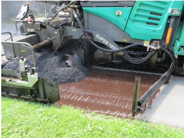
Figure 4.6 Application of a UTBWC (left) (Image credit: A. Braham) and a thin overlay (right) on AC roads (image from RoadResource.org).
