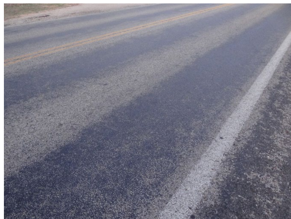
Figure 4.2 Oxidation and raveling (left), and bleeding (right) on asphalt concrete roads. (Image credit: RoadResource.org.)
