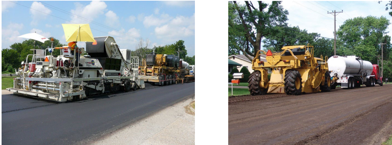
Figure 4.8 Application of HIR (left) and FDR (right) (image from RoadResource.org.)
