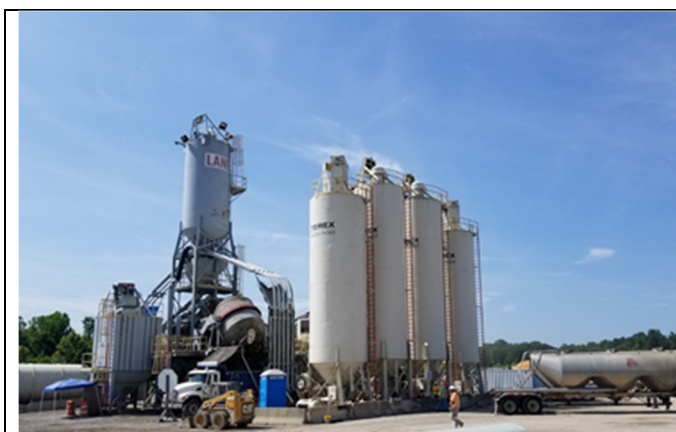
Figure 47 Batch plant used by contractor to produce mainline paving mixture included in PEM pilot project.
