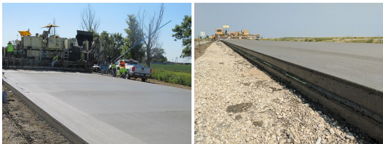
Figure 17 Overall view pavement slab behind paver—Harrison I-29 (2020).
