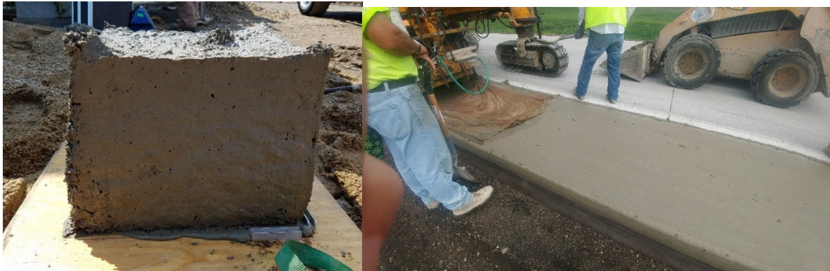
Figure 3 Box Test PEM shoulder mix and paving.
