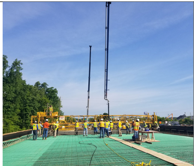
Figure 50 SAM tests performed at bridge deck concrete placement.
