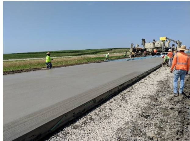
Figure 2 Cedar Valley Paving on US 20.
