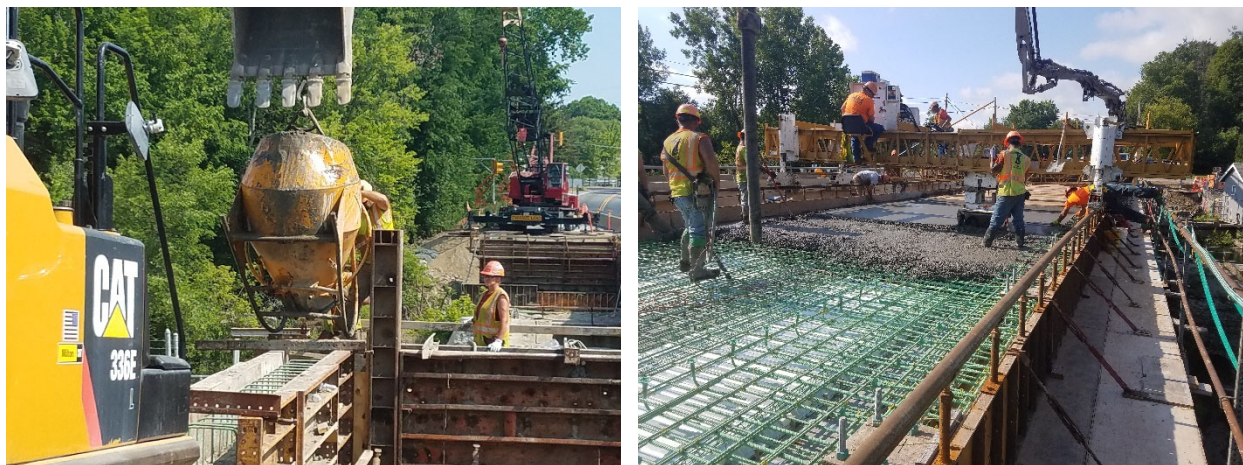
Figure 44 Typical concrete placements on-site.
