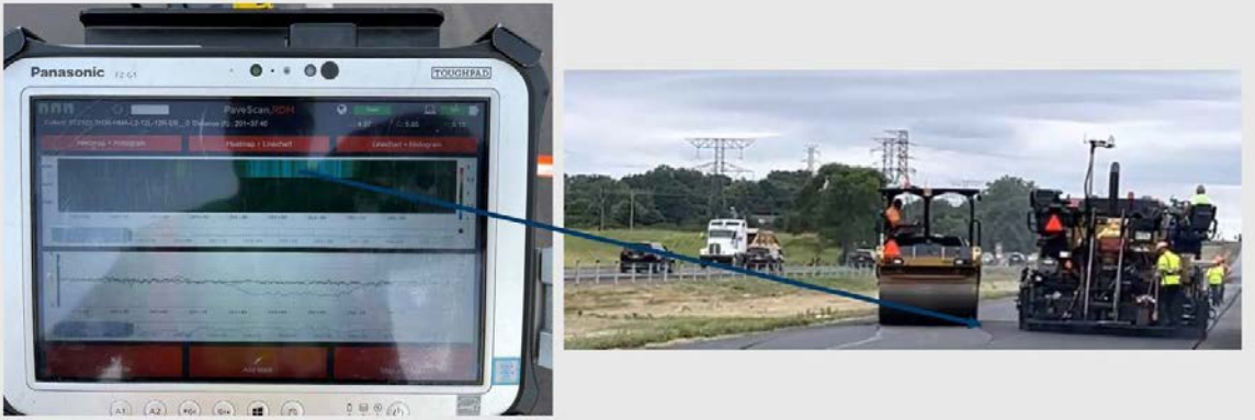
FIGURE 35 Low density area corresponding to roller direction change locations.
