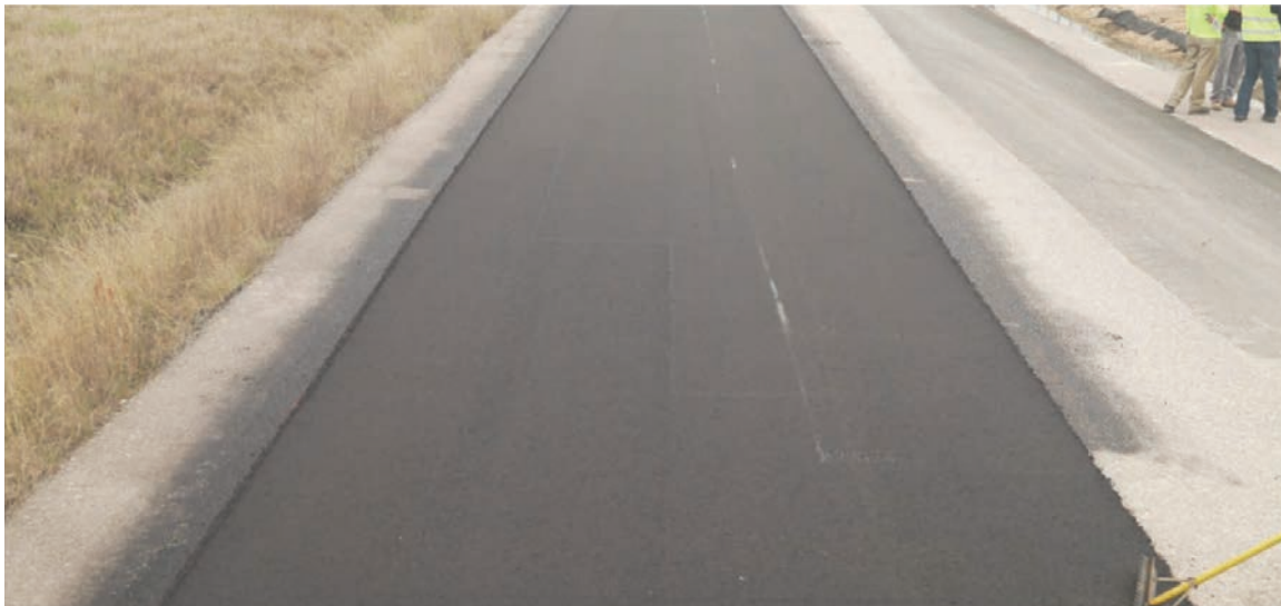
FIGURE 17 January 2019 photo of partially completed project in Freeport, Texas.
