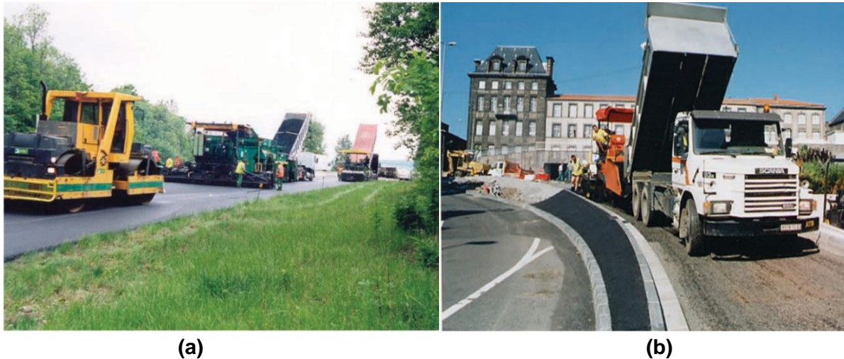
FIGURE 1 Photographs of HMAC projects in France: (a) A-31 Highway, Toul-Langres, France (150 mi slow and lanes, 270,000 tons rPE HMAC base course) and (b) Tramway Lane, Clermont-Ferrand, France (heavy-duty rPE HMAC wearing course).
