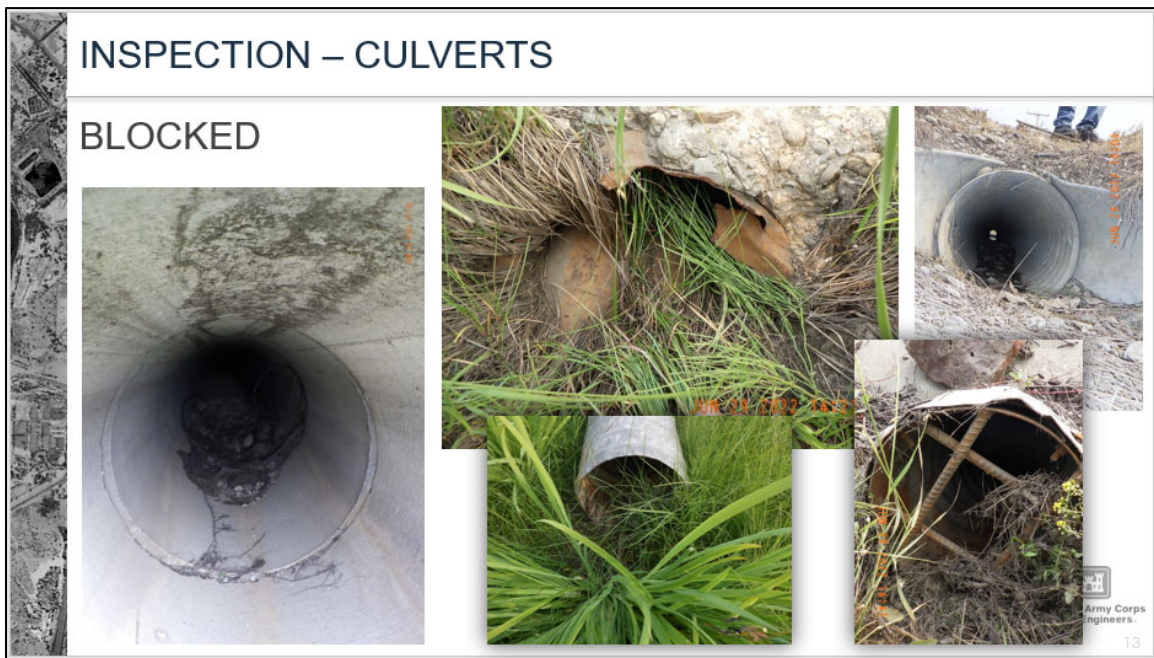
FIGURE 5 Photos of culverts.
