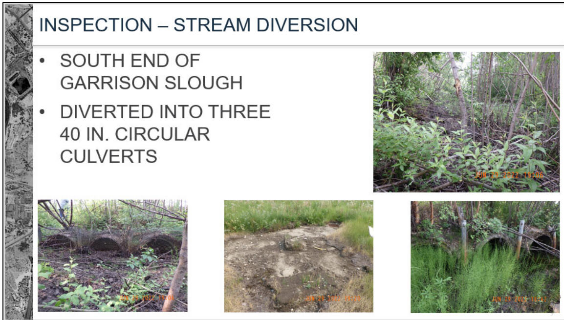
FIGURE 4 Photos of stream diversion.
