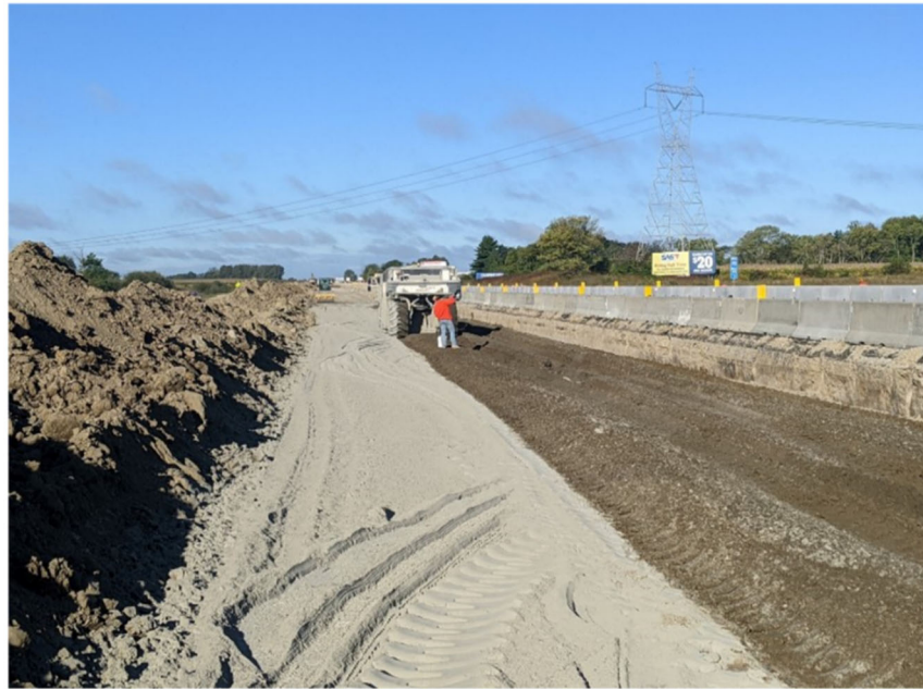
FIGURE 1 Cement added to stabilize subgrade.
