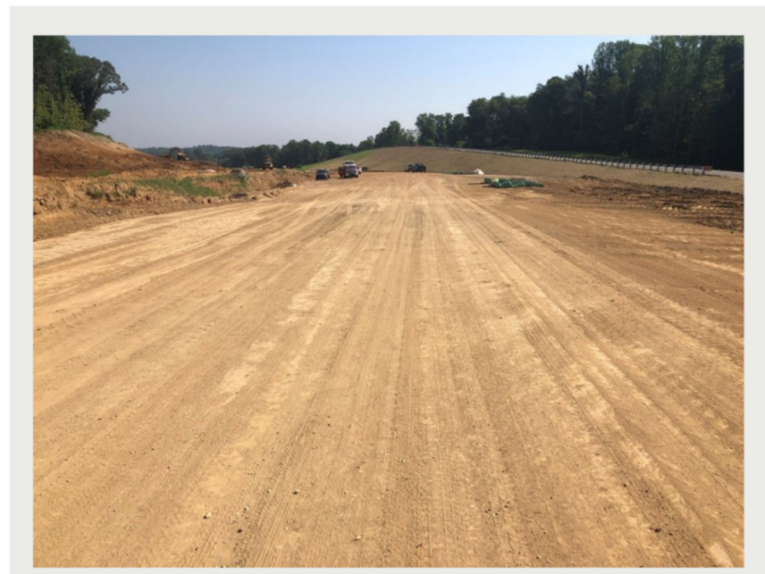
FIGURE 2 Fully compacted cement-stabilized subgrade.
