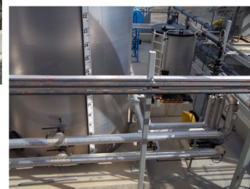
FIGURE 11 Potential effect of binder residual line fill on binder quality.
