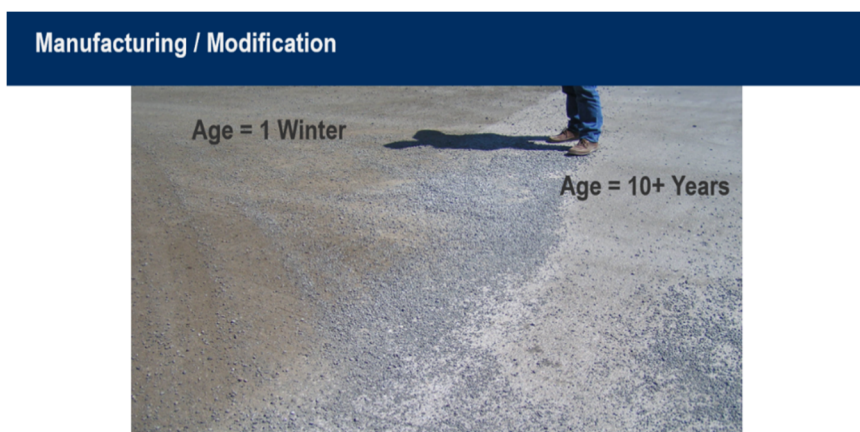
FIGURE 13 Stripping of less than 1-year-old asphalt pavement.
