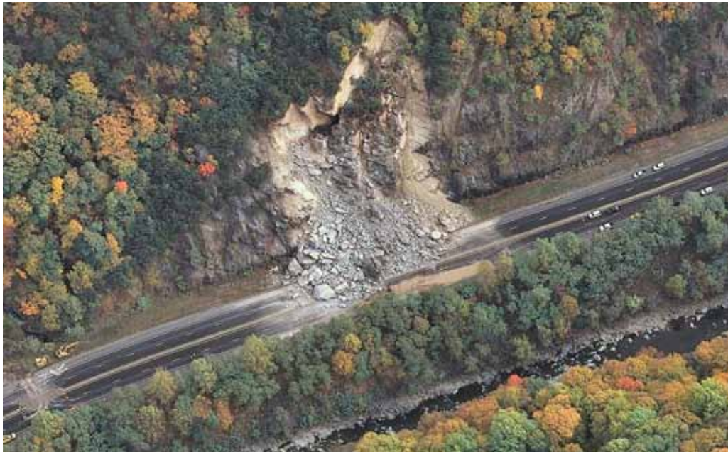
A rockslide in October 2009 closed Interstate 40 in North Carolina for nearly six months. (Photograph: North Carolina Department of Transportation)
