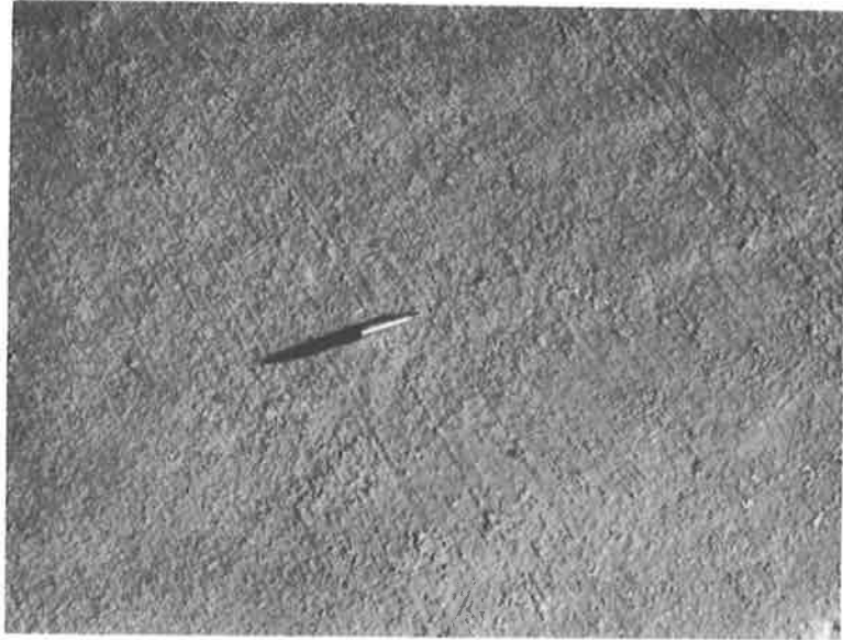
Figure 8. Final surface texture of broomed mortar section.
