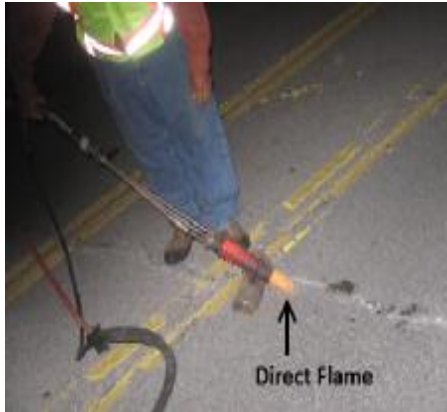
FIGURE 14: Current hot air blasting process.
