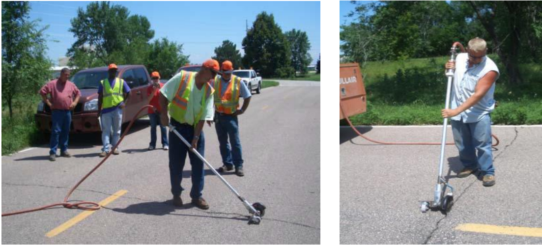
FIGURE 5: First regional panel field test and demonstration.
