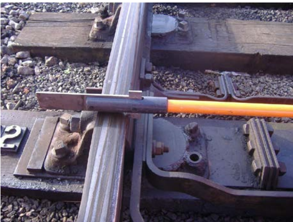
Figure 4C: Switch Gauge 2 used to inspect for switch rail damage.
