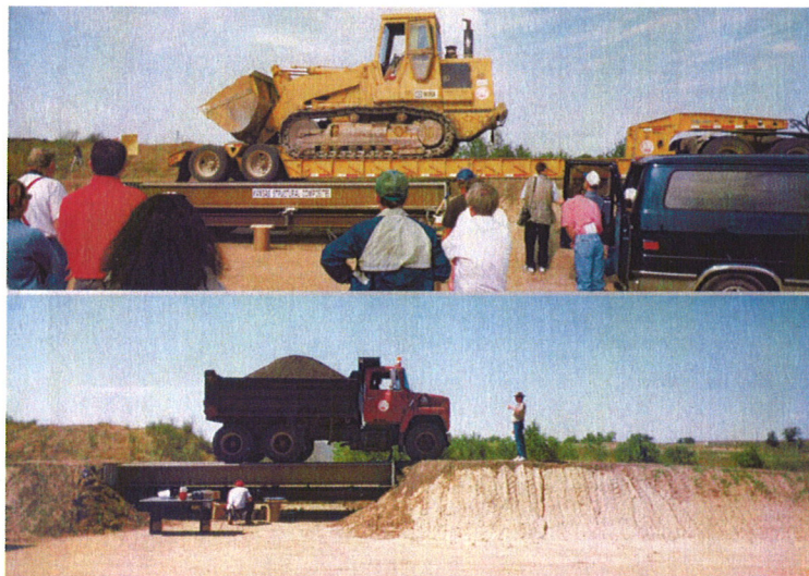
No-Name Creek Bridge with FRP composite decks under test in Russell, Kansas
