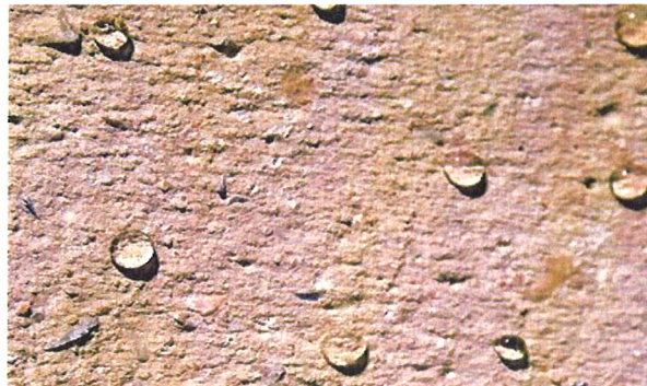
Waterproofing concrete with Hycrete
