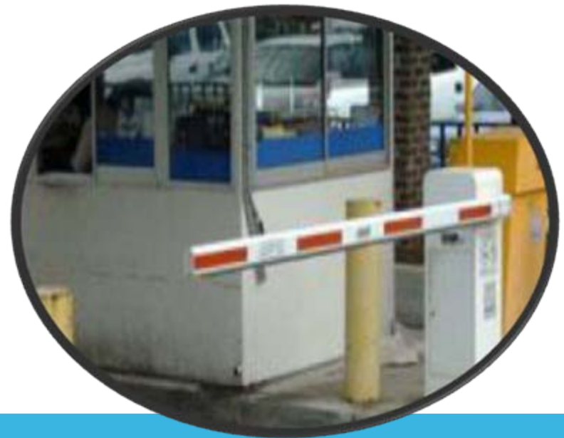
CHAPTER 3: FIGURE 29: Token-based Drop Arm Barrier System
