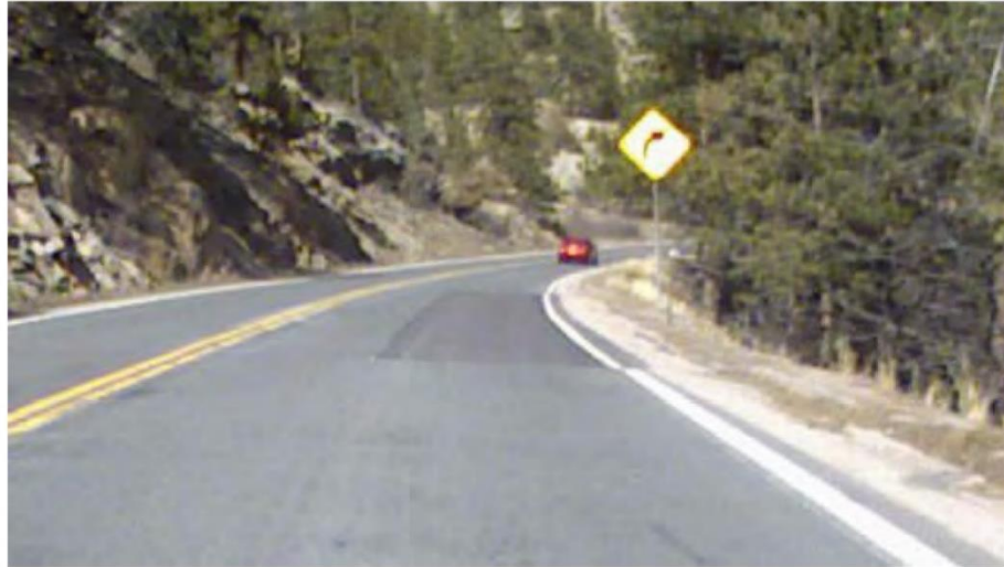
Figure 12 -MP 65.16, Completed pavement and embankment repair section.
