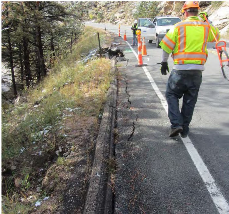
Figure 10 - MP 65.17, Facing south, Damaged asphalt curb, paved shoulder and embankment slope.
