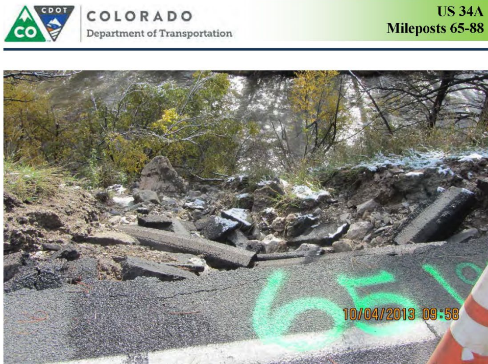
Figure 11 - MP 65.17, Facing east, Washed out embankment and undermined asphalt curb and pavement.
