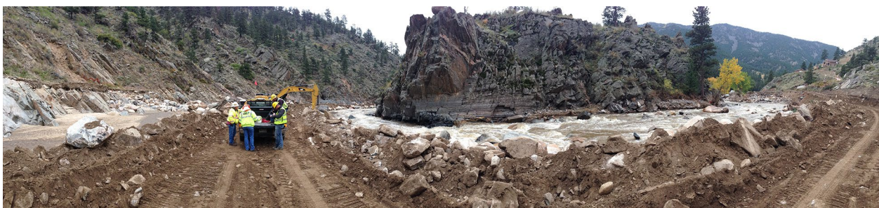
Figure 1-3: Temporary repairs on U.S. 34 following the 2013 Colorado Flood (CDOT, used with permission)
