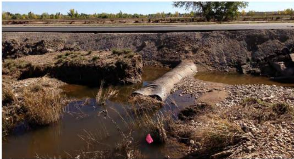
Figure 27 - MP 62.8, Facing South, Scour and damaged CMP
