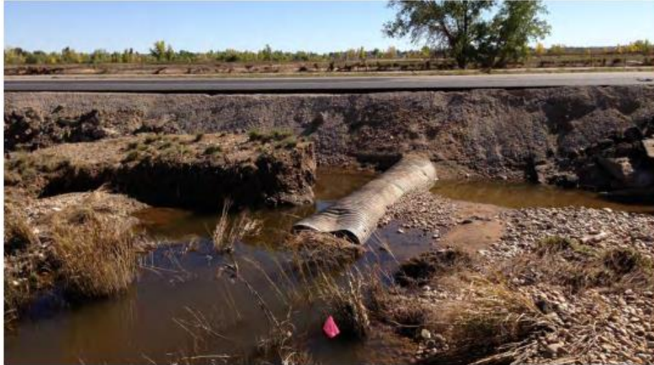
Figure 13 - MP 62.10, Facing south, Damaged 18 inch corrugated metal pipe (CMP)
