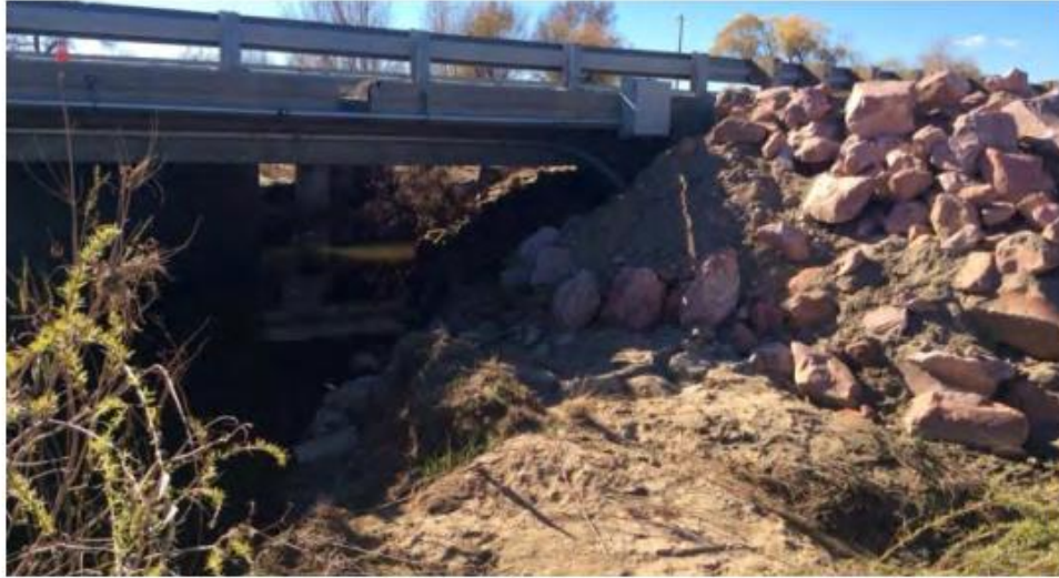
Figure 22 - MP 62.09, Facing south, Repaired west abutment on the north side of Structure D-16-CG.
