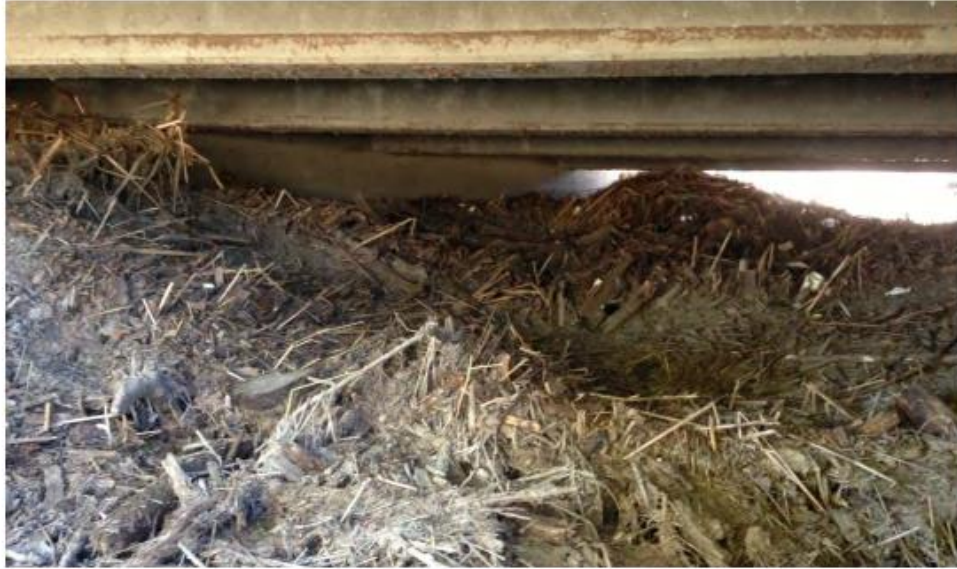
Figure 15 - MP 62.09, Structure D-16-CG, Debris underneath bridge structure
