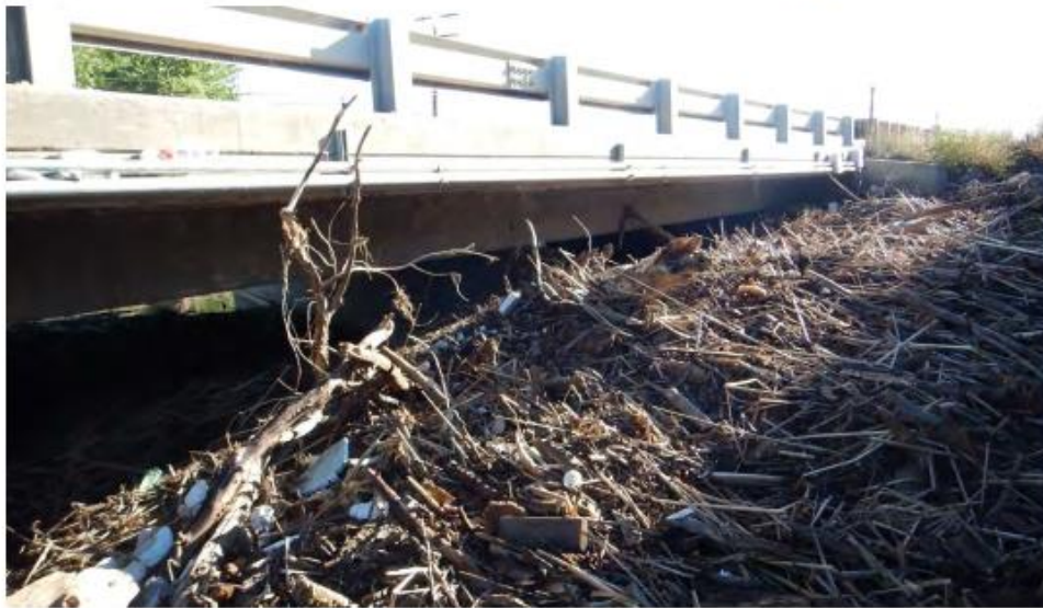
Figure 18 - MP 62.09, Structure D-16-CG, Debris up to the structure
