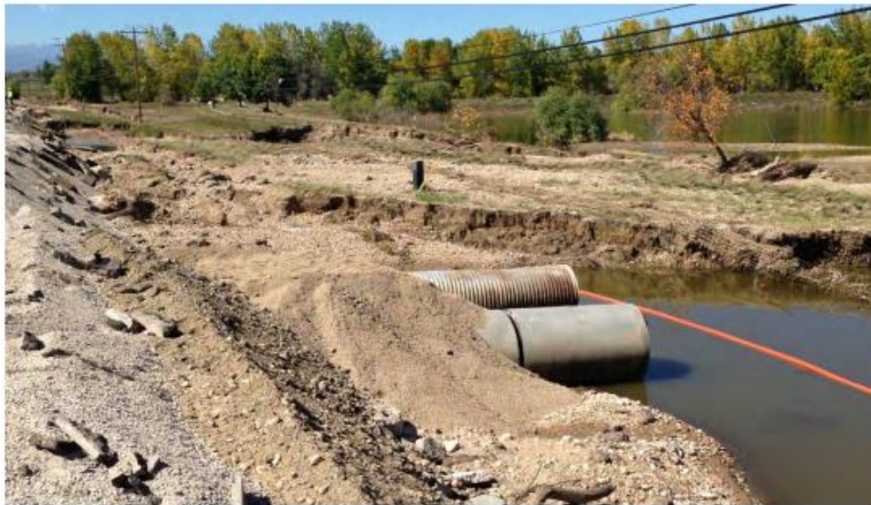
Figure 12 - MP 62.18, Facing west, Damaged twin culverts into gravel pond north of SH 119
