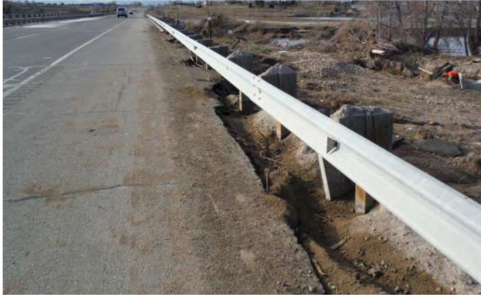
Figure 17 - MP 62.09, Structure D-16-CG: Roadway erosion at northeast approach rail
