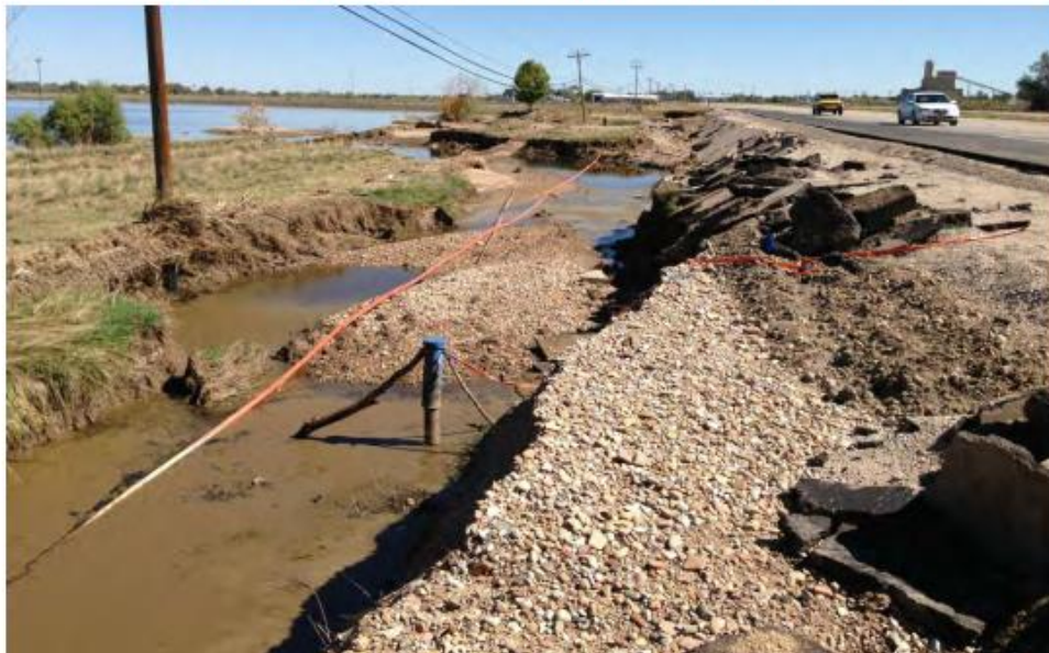
Figure 14 - MP 62.18, Facing east, Scour, embankment damage and exposed utilities
