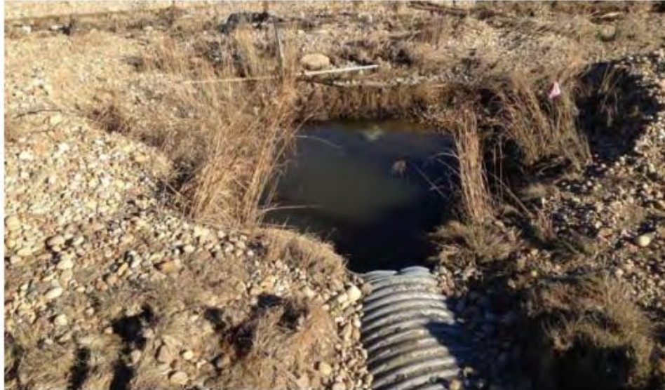
Figure 28 - MP 62.93, Facing north, Scour hole and damage to CMP culvert north side of SH 119
