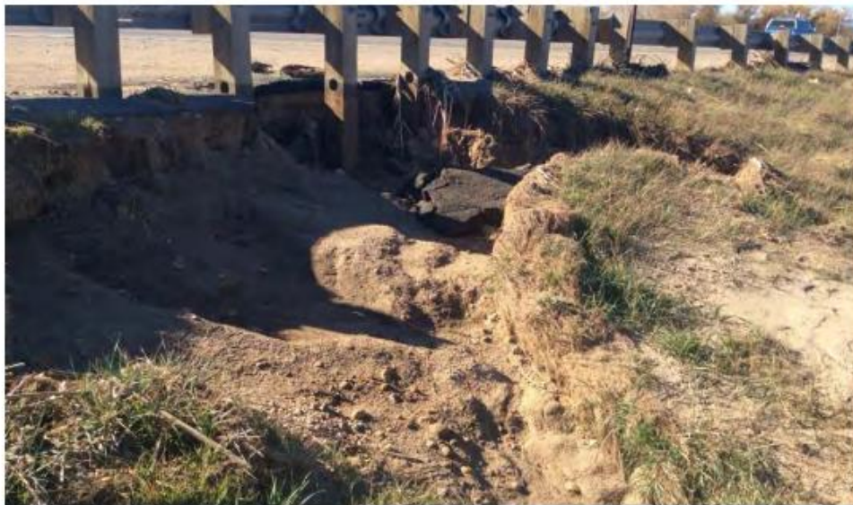
Figure 20 - MP 62.09, Structure D-16-CG, Erosion at approach
