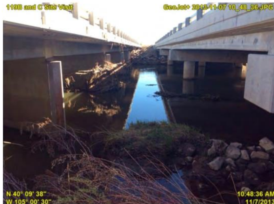
Figure 10 - MP 62.03, Facing East, Debris on south side of Structure D-16-CG to the north of Structure D-16-DR
