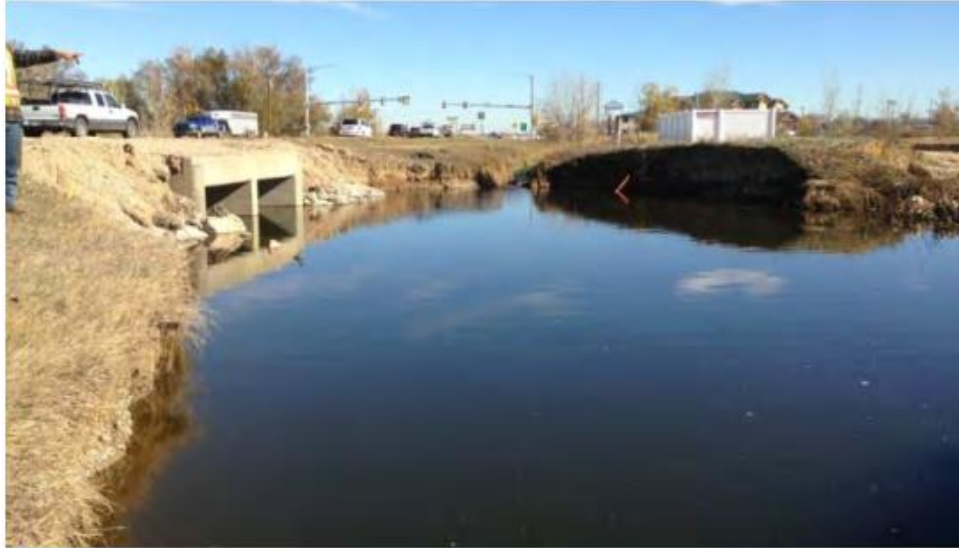
Figure 30 - MP 63.03, Facing East, Scour hole at the inlet of the double 9 ft x 5 ft CBC, south side of SH 119.
