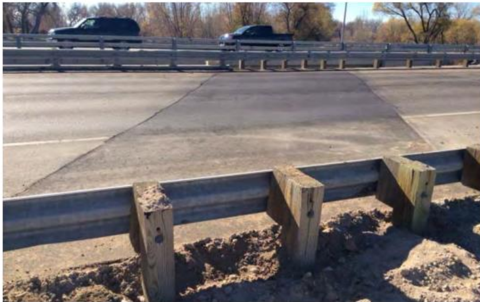
Figure 23 - MP 62.03, Facing south, Repaired roadway section at west abutment on Structure D-16-CG
