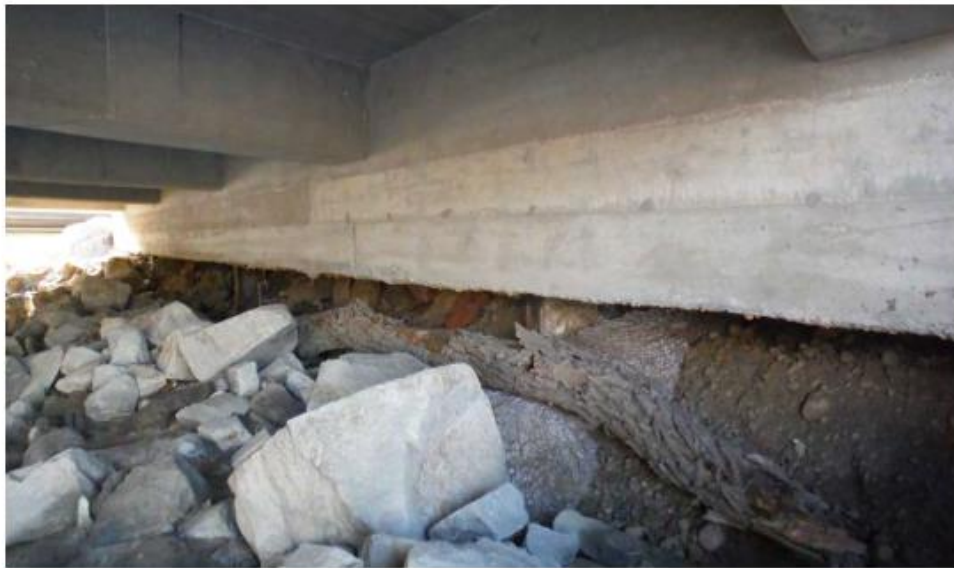
Figure 16 - MP 62.09, Structure D-16-CG, Exposed piles at west abutment
