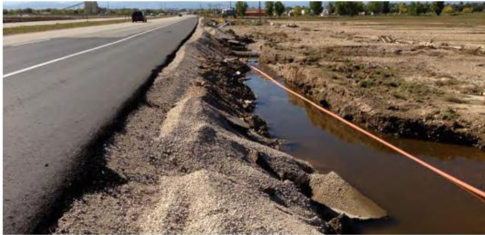
Figure 32 - MP 62.8, Facing west, Repaired roadway shoulder and partial repair of embankment north of SH 119
