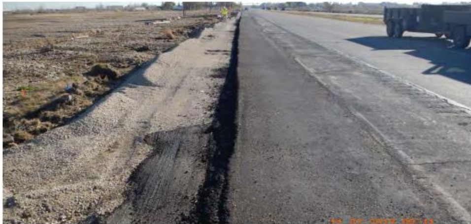
Figure 33 - MP 62.8, Facing west. Repaired roadway shoulder and partial repair of embankment north of SH 119
