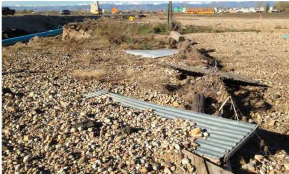
Figure 31 - MP 62.83, Facing west, Deposited roadway embankment material and damaged ROW fence north of SH 119
