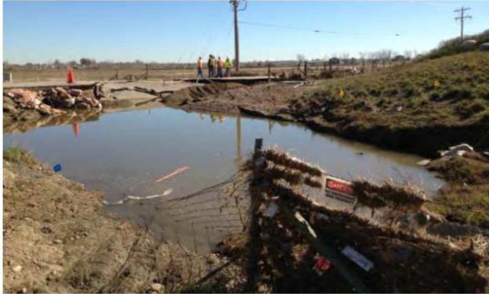
Figure 11 - MP 62.52, Damage to roadway drainage, ditch and embankment at WCR 7 intersection south of SH 119, facing East
