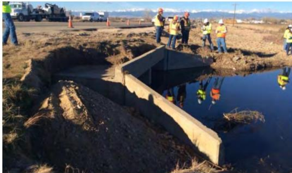
Figure 29 - MP 63.03, Facing West, Scour hole and damage at headwall and wingwalls at outlet of double 9 ft x 5 ft CBC, north side of SH 119.
