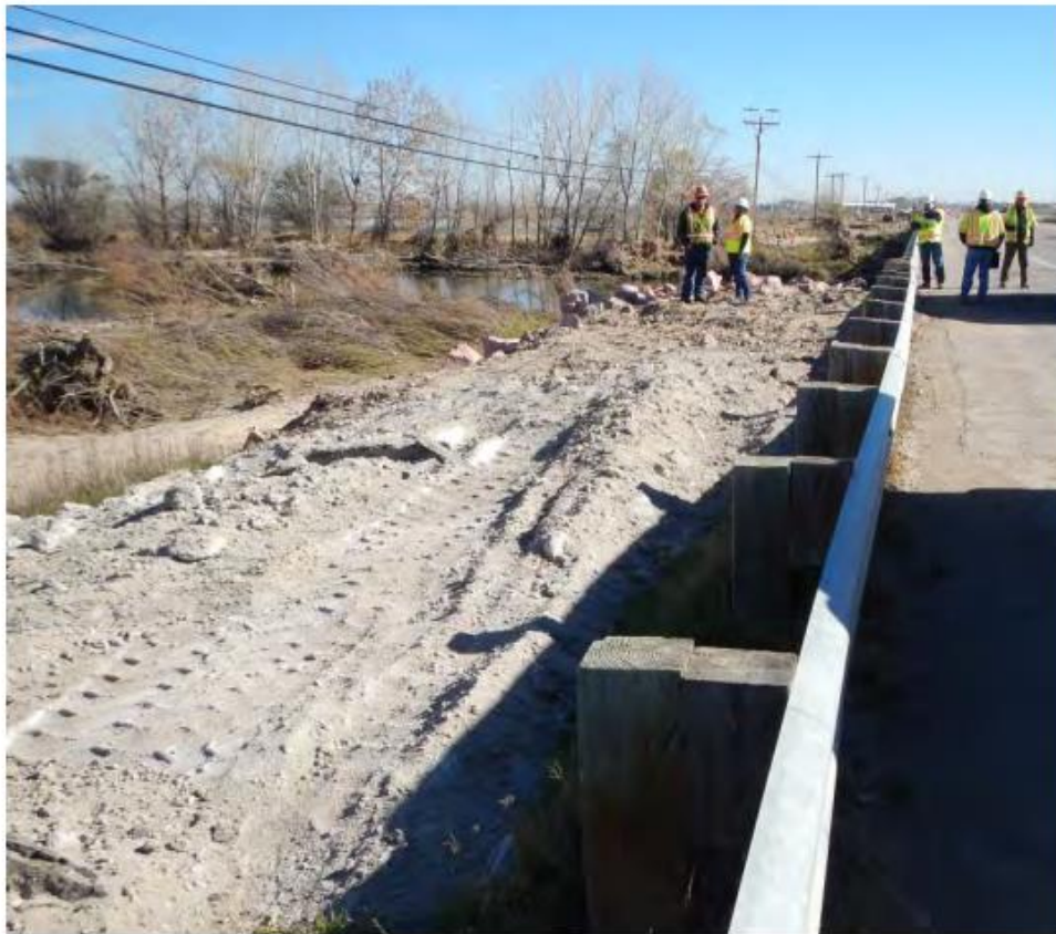
Figure 21 - MP 62.09, Facing east, Repaired embankment at Structure C-16-CG on the north side of SH 119 (looking east)
