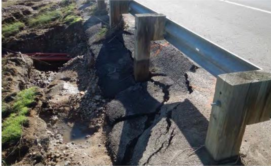
Figure 19 - MP 62.09, Structure D-16-CG, Erosion at approach
